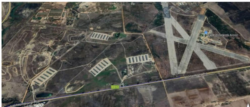
Figure 25: The development will also require a potable water pipeline to be extended eastwards from Durbanville by the CoCT along the R312. It will exceed 300m in length but will have no impact on heritage resources as it will be sub-surface in the R312 road reserve.
