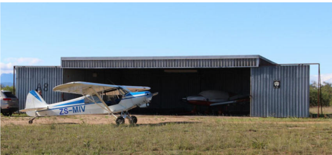
Illustration 8: Hangar built between 1968 and 1980 (Structure # 6; SSTownsend, 15 June 2020)
