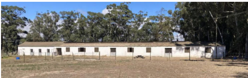
Figure 18: Stables also of concrete blocks with roofs of asbestos sheeting
