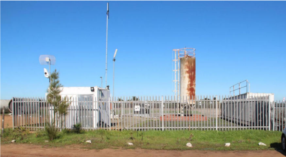
Illustration 9: Miscellaneous service structures, all post 1980 (SSTownsend, 15 June 2020)
