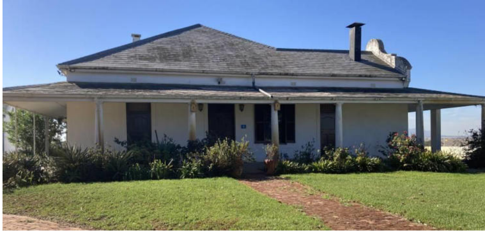
Figure 22: The roof is of asbestos cement shingles and the veranda roof is supported on steel pipe columns, Pre-cast concrete columns and brick columns
