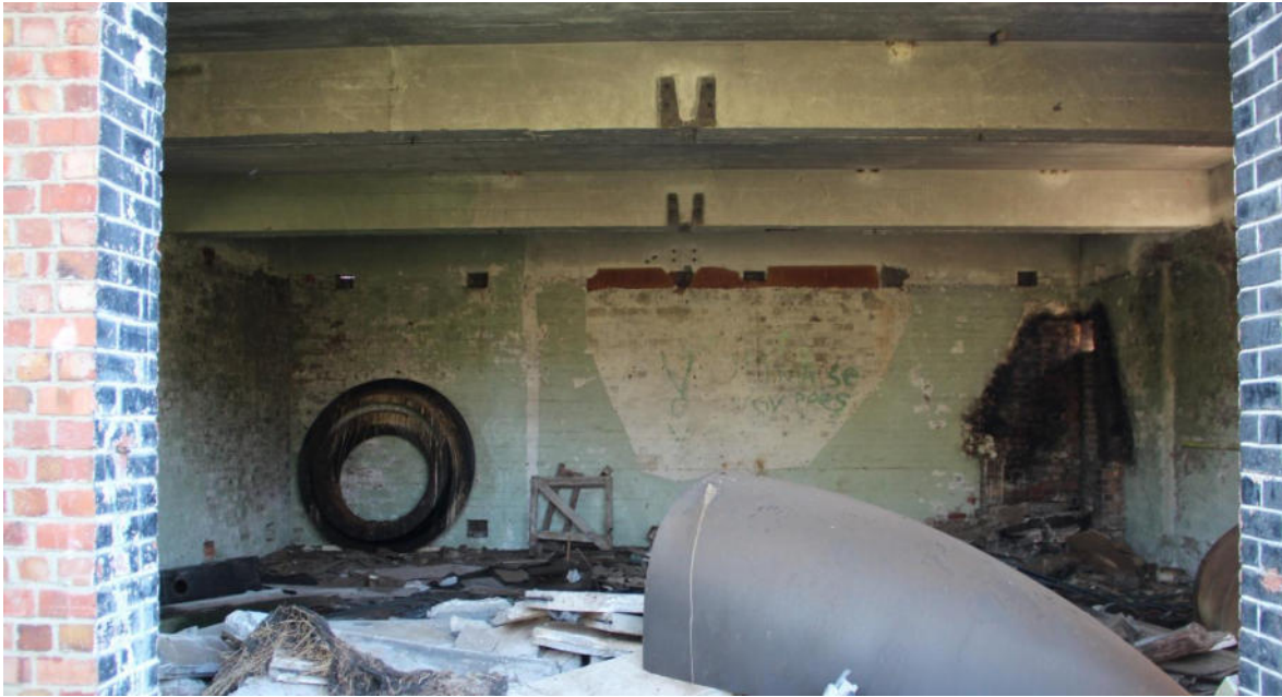
Illustration 17: The interior of the Workshop showing the evidence of a gantry and a forge (Structure #2, SSTownsend, 15 June 2020)
