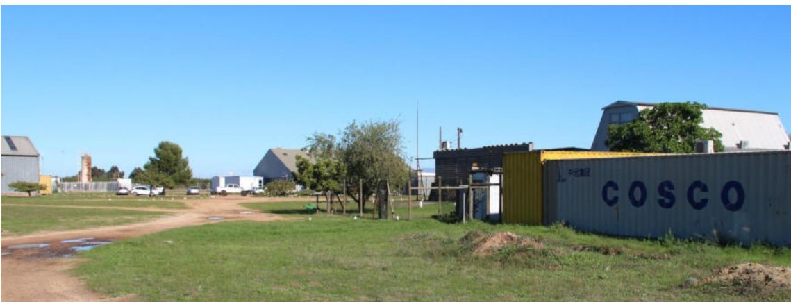
Illustration 5: View towards the Flying School building at the centre (Structure # 11; SSTownsend, 15 June 2020)
