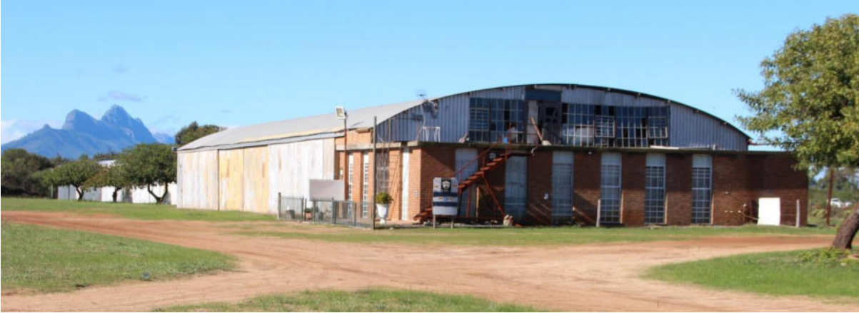
Illustration 3: Hangar built in three distinct phases after 1980 (Structure # 10; SSTownsend, 15 June 2020)
