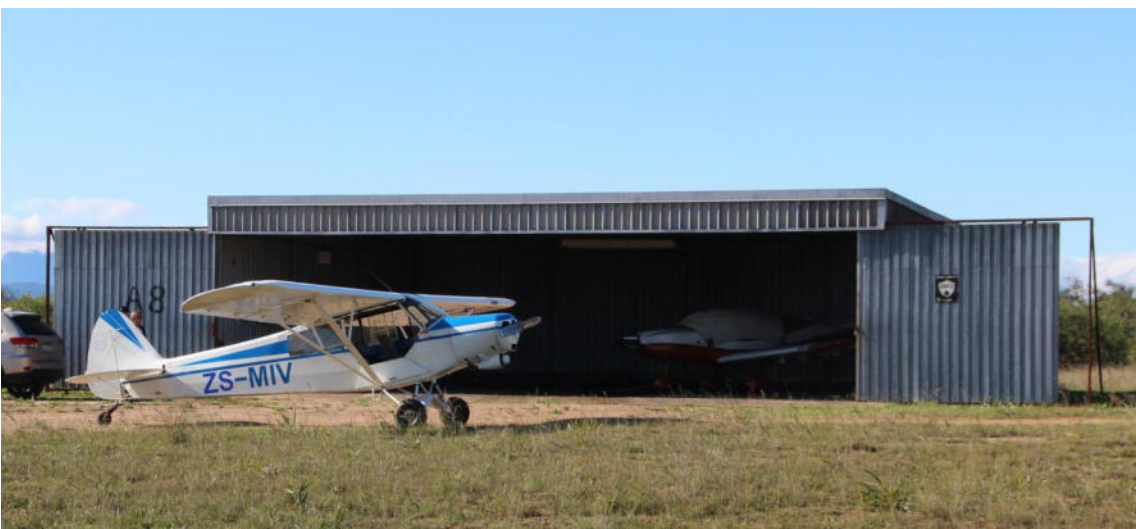
Illustration 8: Hangar built between 1968 and 1980 (Structure # 6; SSTownsend, 15 June 2020)
