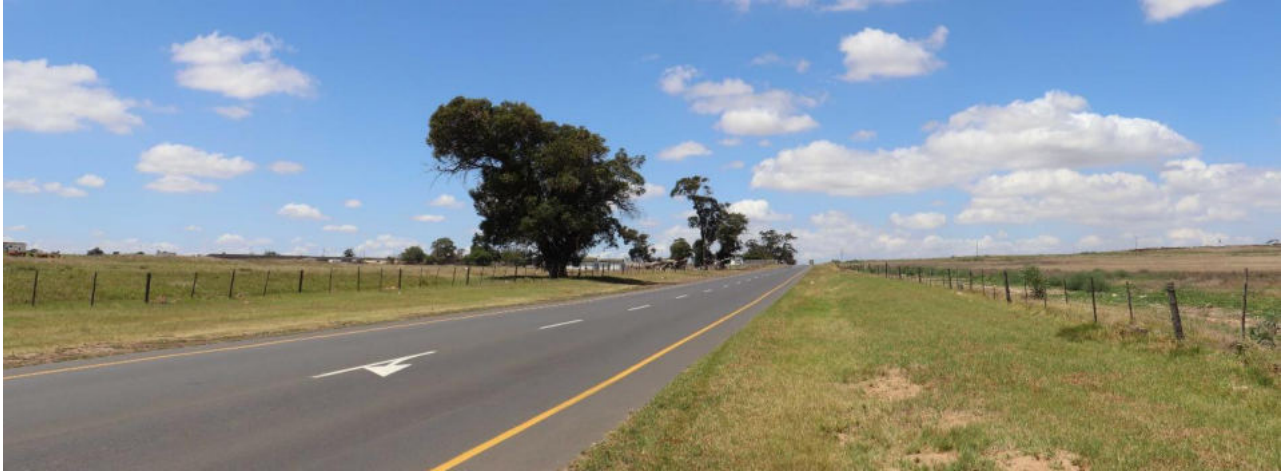
Figure 91: Visibility testing – view from 900m away from the site, looking north east along the R312. (Smit, 2022)
