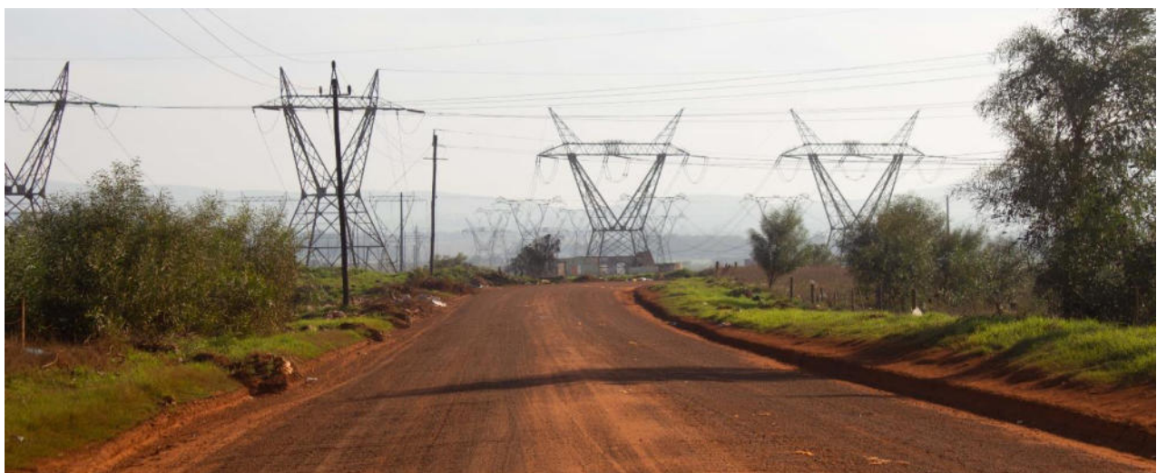
Figure 40: Site photograph demonstrating the intensity of visual clutter as a result of the Eskom power lines where these cross Canary Street near Fisantekraal (Smit, 2021)
