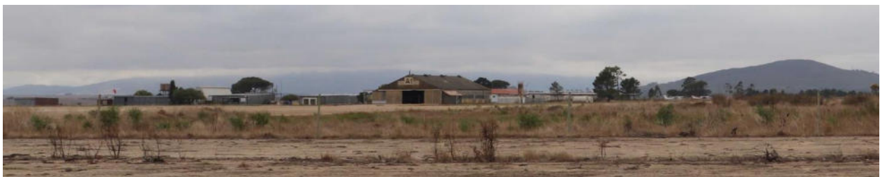
Figure 3: Site visit photograph showing existing structures on site associated with the Cape Winelands Airport (Smit, 2022)
