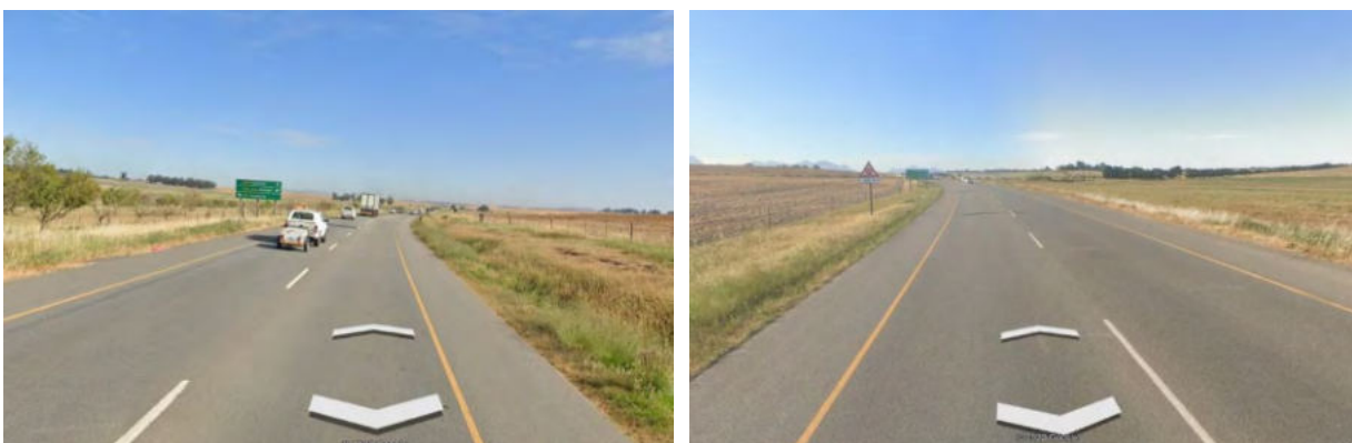
Figure 6: Koelenhof Road (source: Google Earth)
