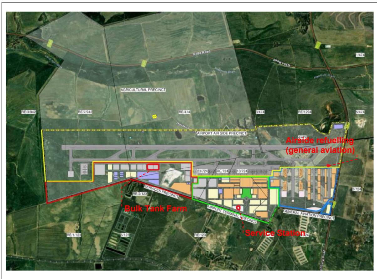
Figure 3.1: Aerial photograph of CWA airport development with proposed location for fuel facilities
