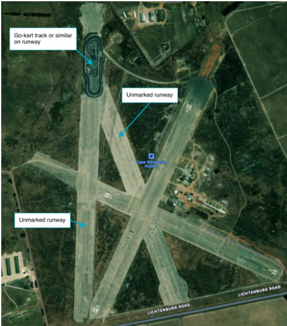
Figure 3.2: Current airfield showing 2 runways in use and 2 derelict runways (one with go-kart track)
