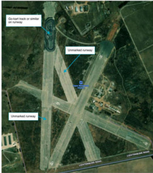
Figure 3.2: Current airfield showing 2 runways in use and 2 derelict runways (one with go-kart track)
