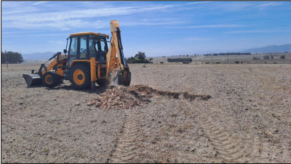
Figure 11: Establishment of soil test pits using the Tractor Loader Backhoe (TLB).
