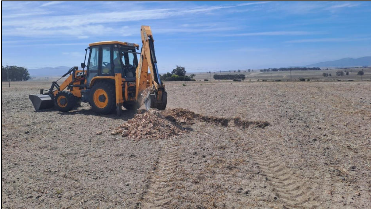
Figure 13: Establishment of soil test pits using the Tractor Loader Backhoe (TLB).
