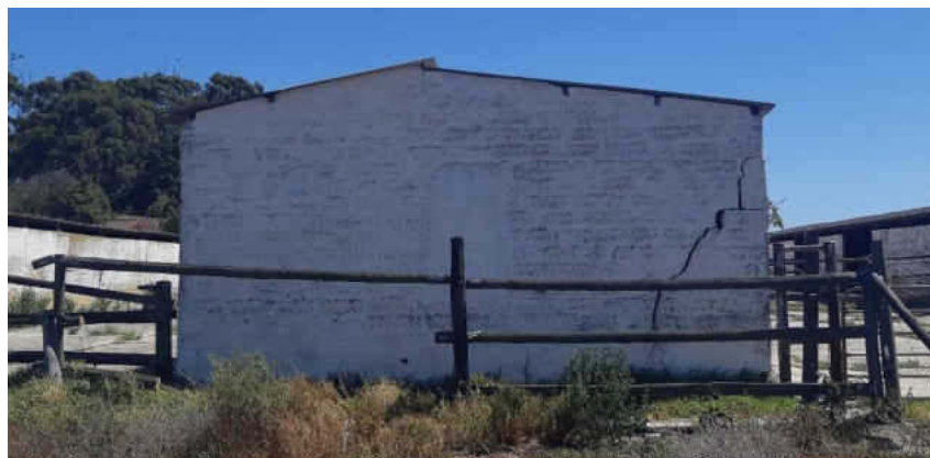
Figure 56: Corner down type crack possibly related to potentially expansive nature of subsoils; stable structure located between TP18 and TP15.
