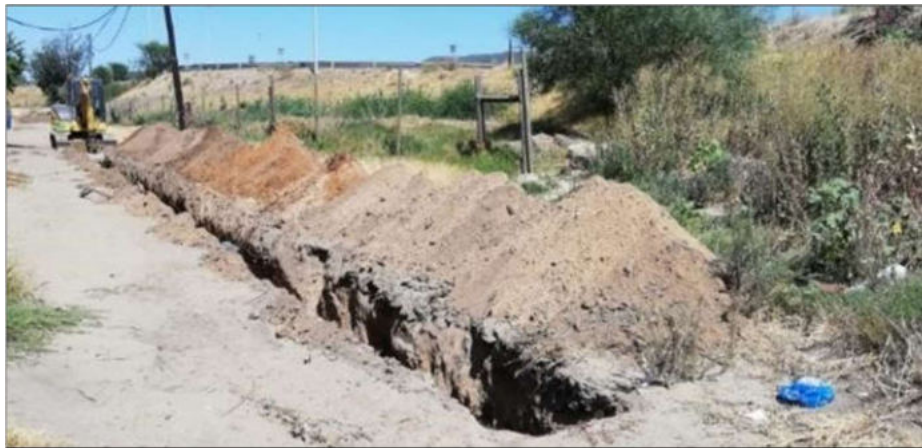
Figure 26: Excavation for trenching with stockpiles alongside.
