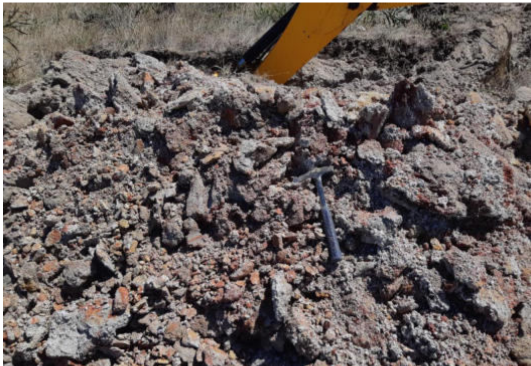
Figure 24: TP04 – Close-up of sandy clayey silt spoil.
