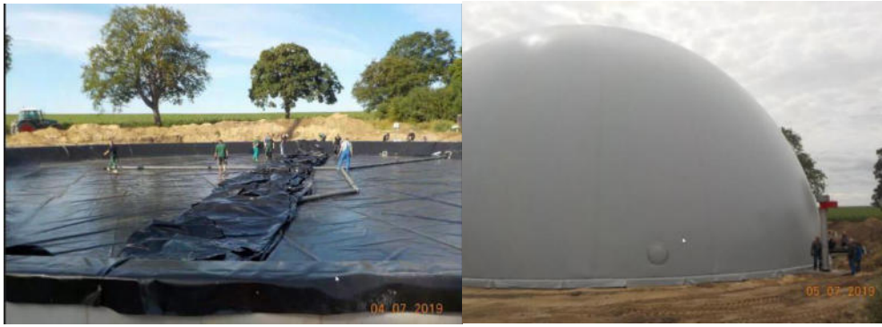
Biogas Bladder Storage
