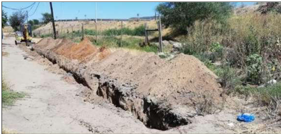
Figure 26: Excavation for trenching with stockpiles alongside.
