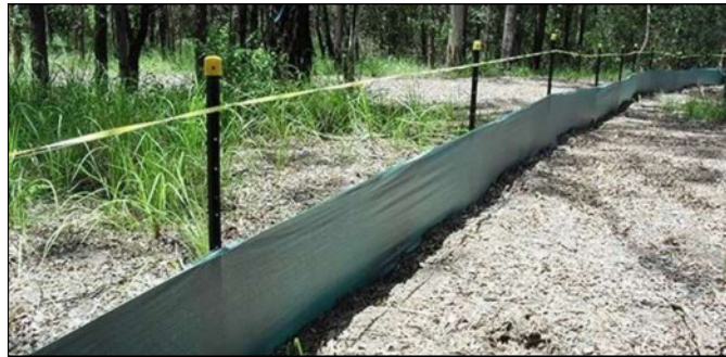
Figure 25: Example of a barrier fence used to demarcate the no-go area around the freshwater ecosystems and the 15 m construction conservation buffer.
