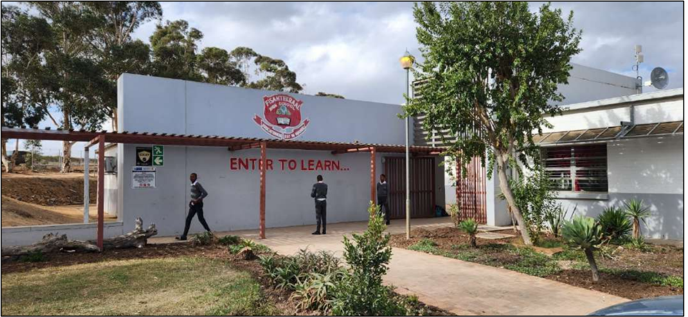
Figure 6: A Site Notice was placed at the Fisantekraal High School.
