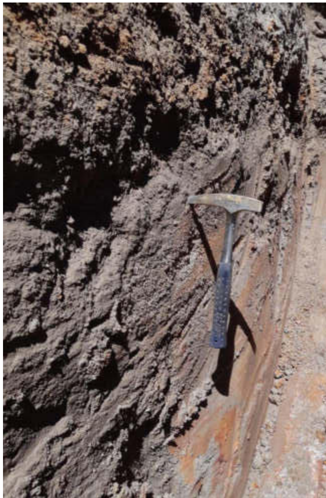
Figure 22: TP04: Close-up of trial pit sidewall. Note cemented nature of nodular ferricrete above hammer, and texture of sidewall ‘smear’ beneath hammer; sand- to clay- dominated with depth.
