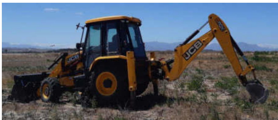
Figure 60: View of JCB 3DX Super Tractor Loader Backhoe excavating a trial pit near the central portion of the site.
