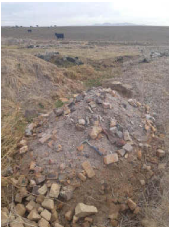
Figure 59: Fill dumped in drainage in northern portion of the site intended for future development.
