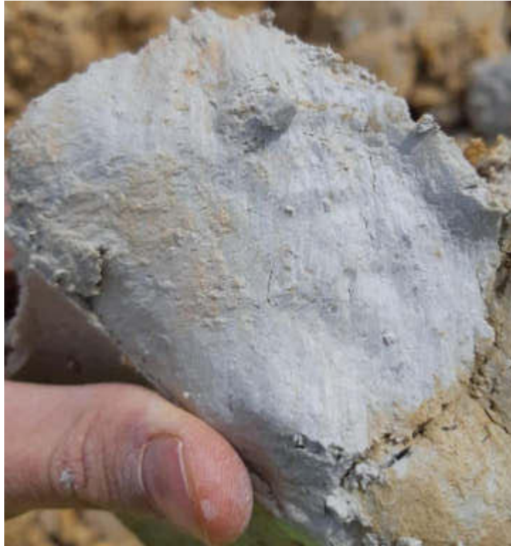
Figure 55: TP44 – Close-up of slightly smoothed/slickensided surface of residual material encountered in trial pit.
