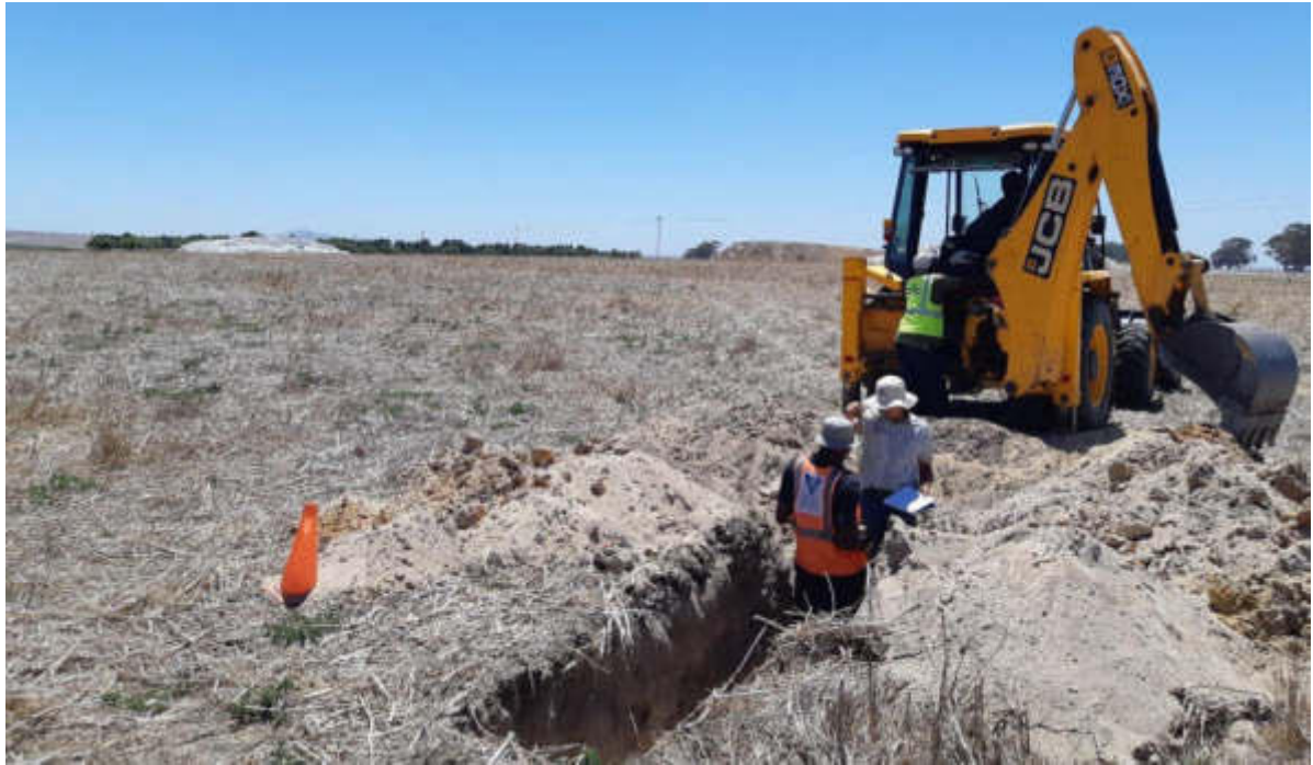
Figure 44: TP21 – GEOSS team conducting DCP test beneath nodular ferricrete horizon. White clay-silt Corrobrick material pictured in the background.
