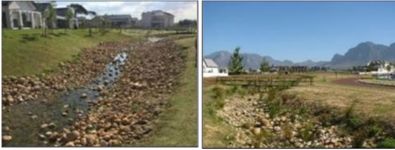
Figure 161: Examples of swales utilised for conveyance of stormwater (FEN: Sept 2024)
