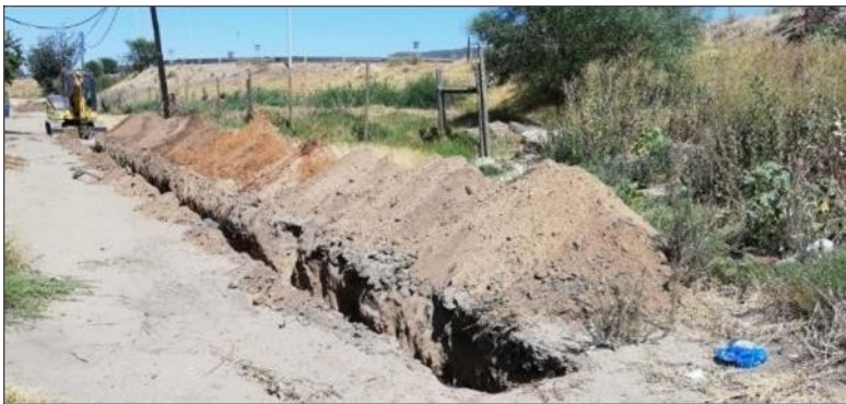
Figure 160: Excavation for trenching with stockpiles alongside (FEN; Sept 2024)
