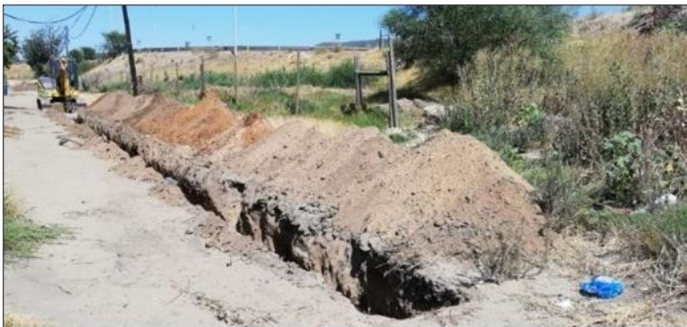
Figure 174: Excavation for trenching with stockpiles alongside (FEN, Freshwater Ecological Assessment, February 2025).
