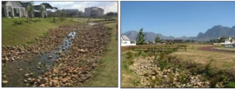
Figure 175: Examples of swales utilised for conveyance of stormwater (FEN, Freshwater Ecological Assessment, February 2025).
