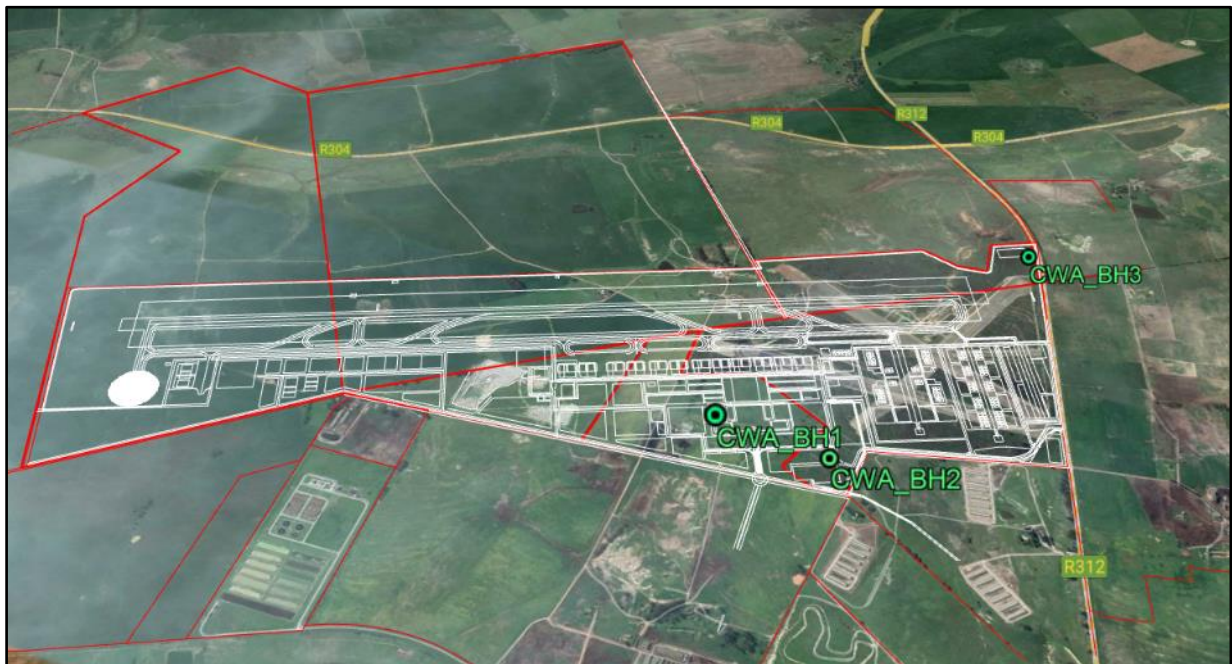
Figure 48: Three production boreholes on site (PHS Consulting, February 2025)
