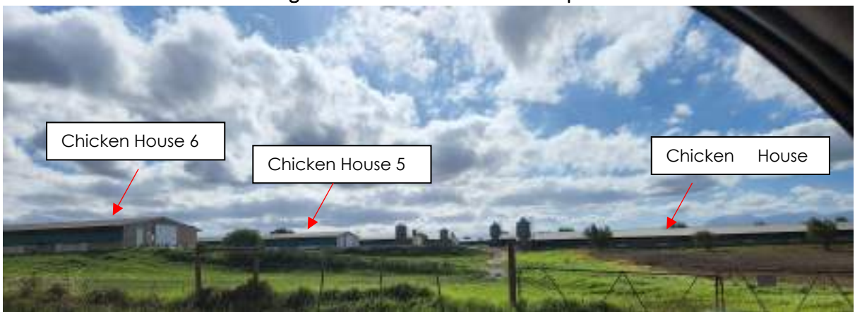
Photo 5: Outside view of chicken house 5, 6 and 10.
