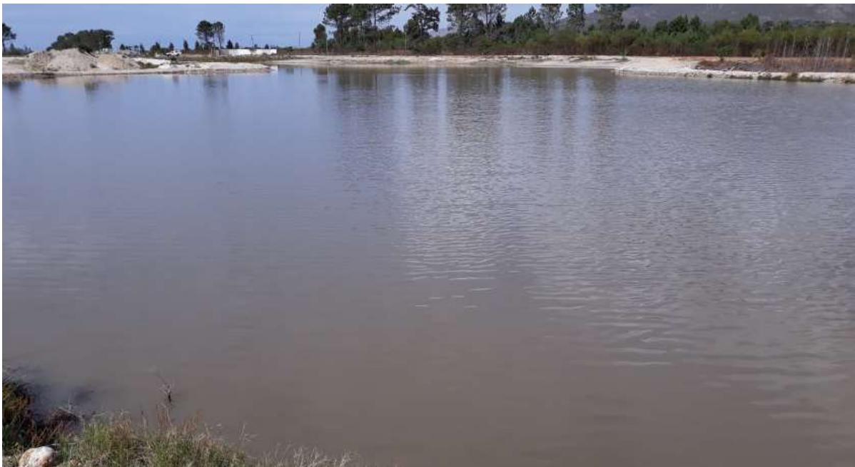
Photo 9: Dam 2 proposed for expansion, surrounded by alien vegetation and bare exposed soil areas.
