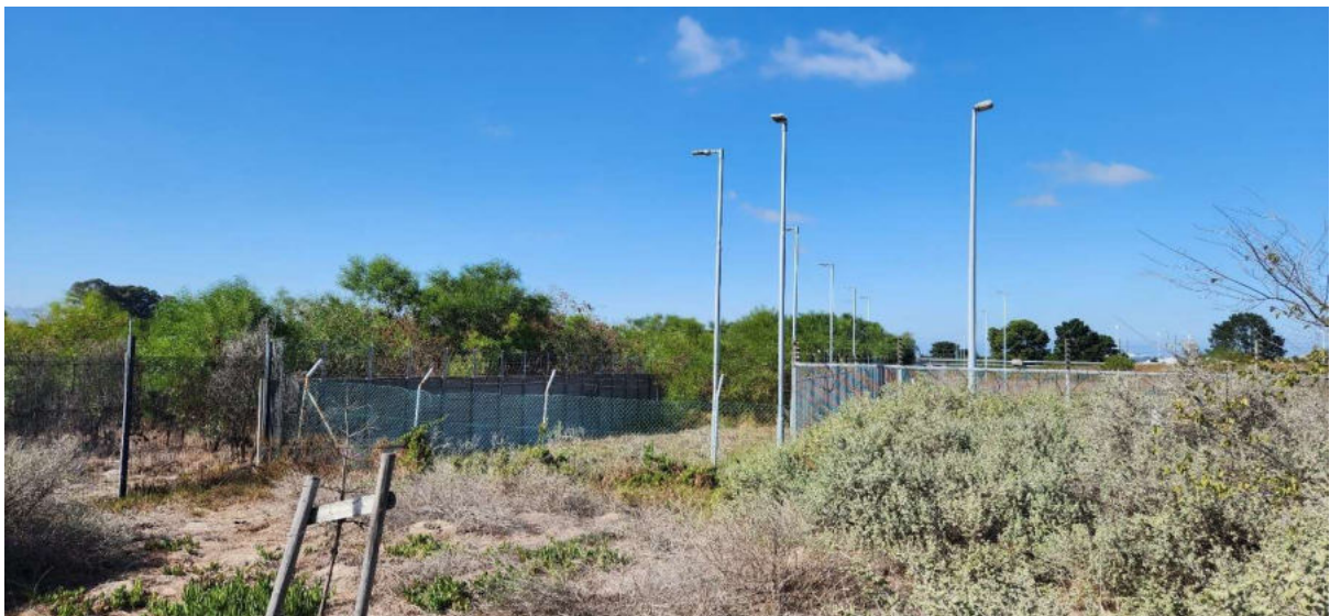
Photo 17: Showing the varied boundary treatments that require attention.
