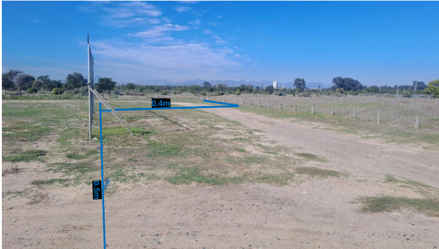
PHOTOGRAPH 12: Area Scanned Showing Utilities Found and Depths – View Looking East
