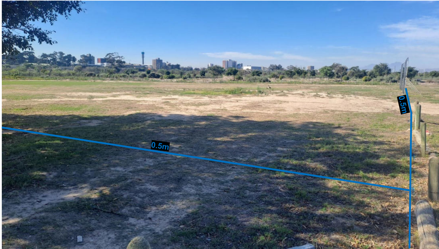
PHOTOGRAPH 11: Area Scanned Showing Utilities Found and Depths – View Looking East
