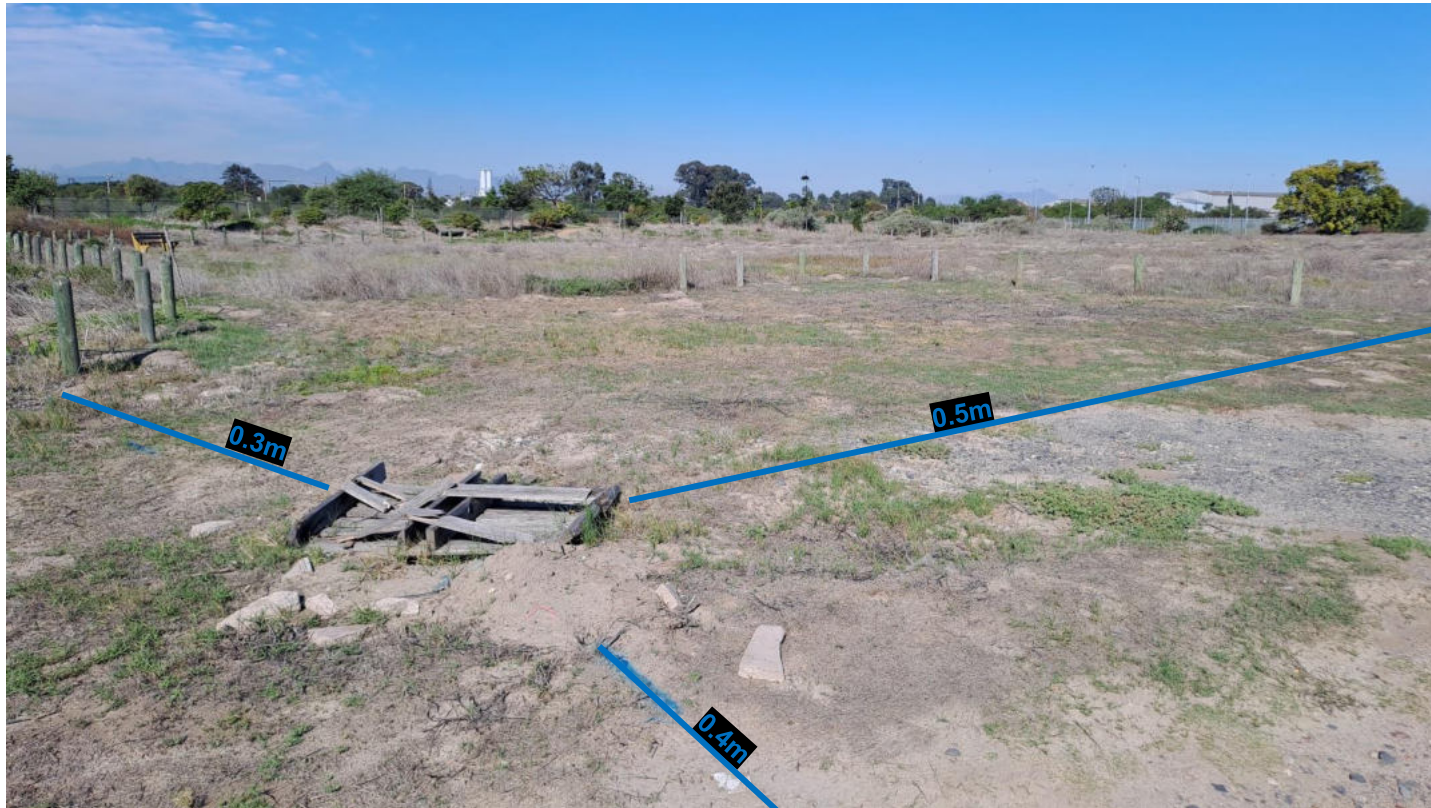
PHOTOGRAPH 14: Area Scanned Showing Utilities Found and Depths – View Looking East
