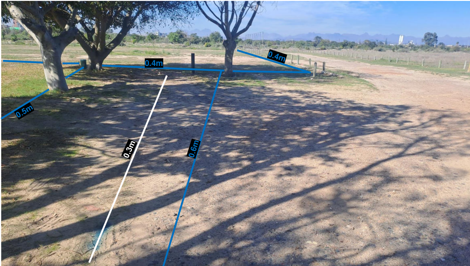
PHOTOGRAPH 10: Area Scanned Showing Utilities Found and Depths – View Looking East
