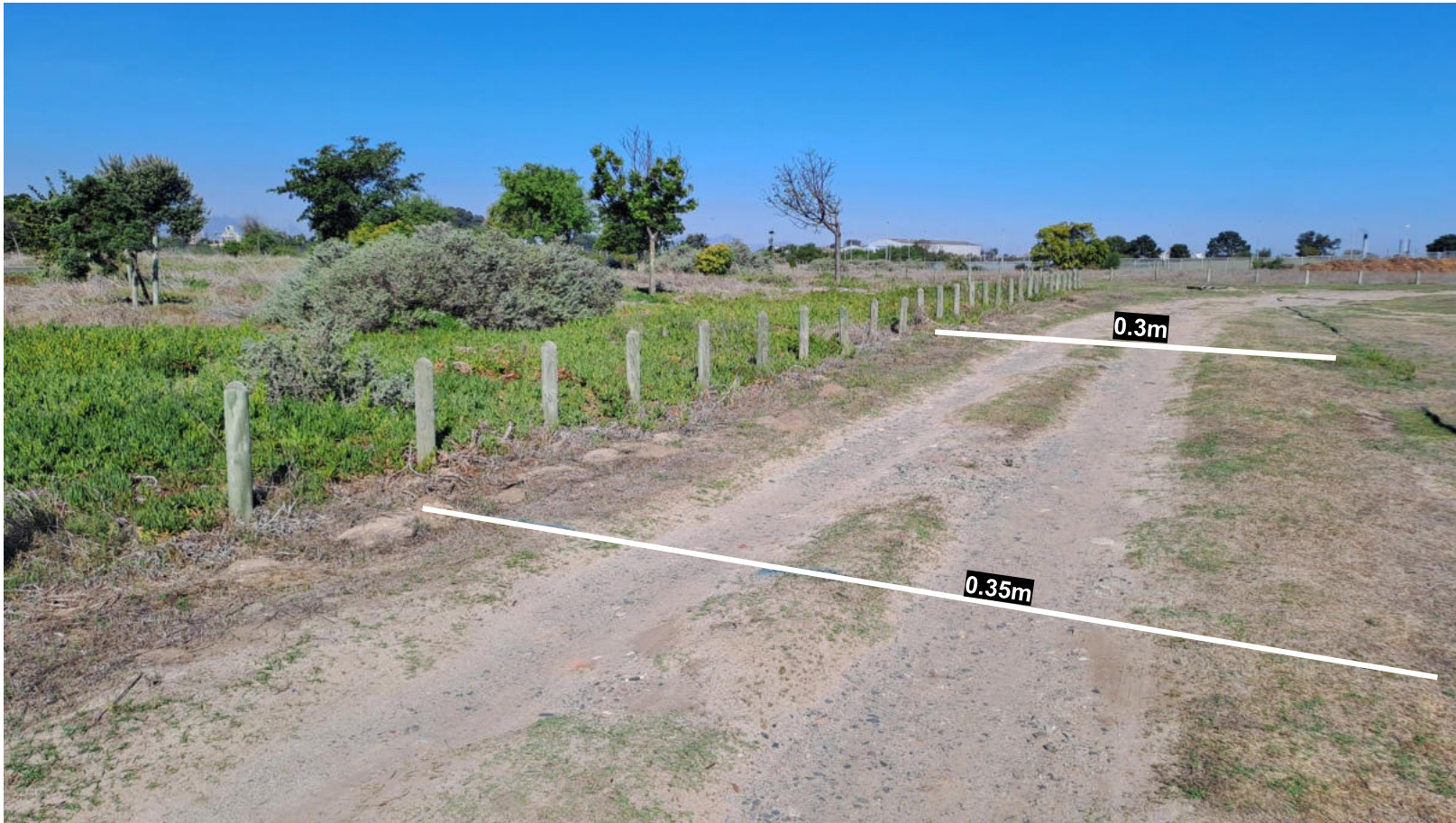
PHOTOGRAPH 15: Area Scanned Showing Utilities Found and Depths – View Looking South – East
