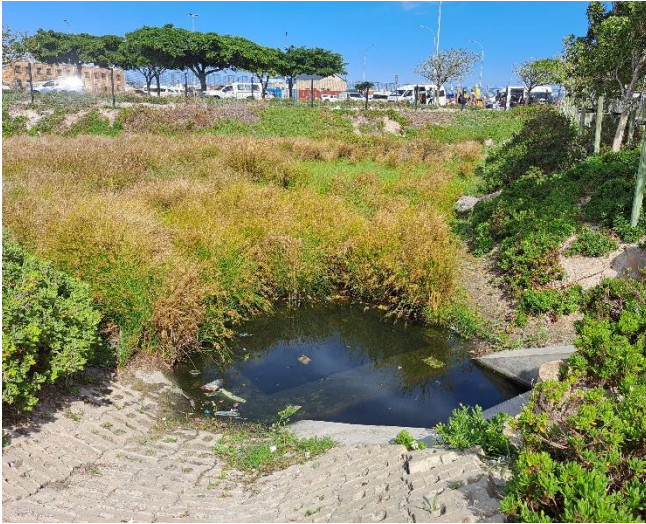
Figure 16. An example of stilling basin, with vegetation downstream, similar to that which is recommended in this report. (Photograph credit: Kate Snaddon)
