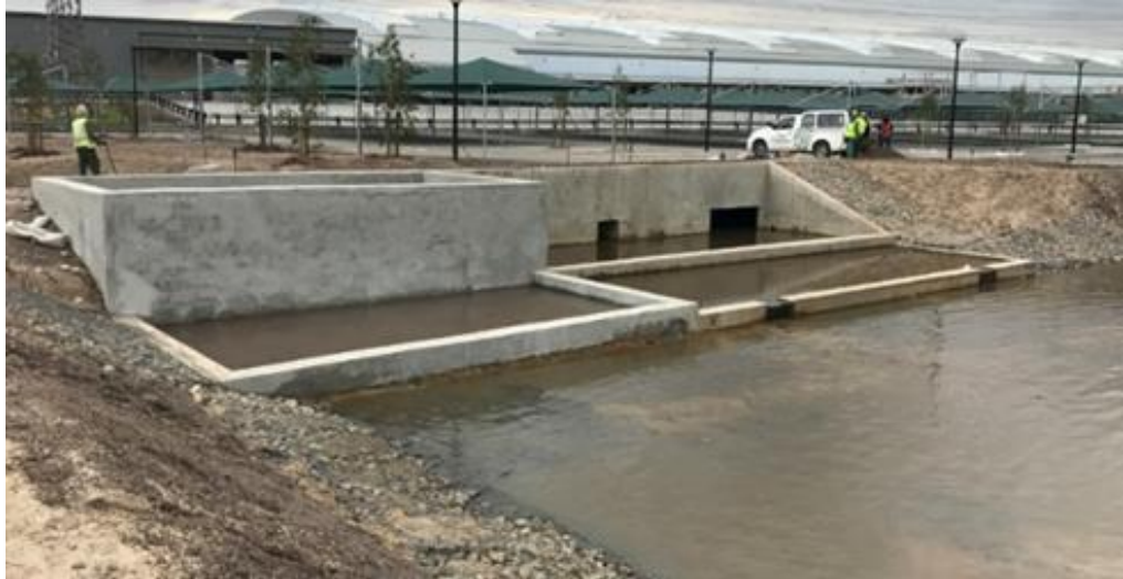
Figure 7: Proposed Stilling Basin Dam Inlet
