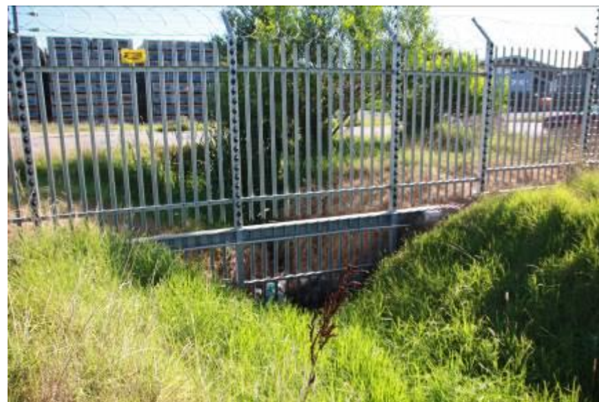
Figure 5b: Storm water drain 2 at southern fence
