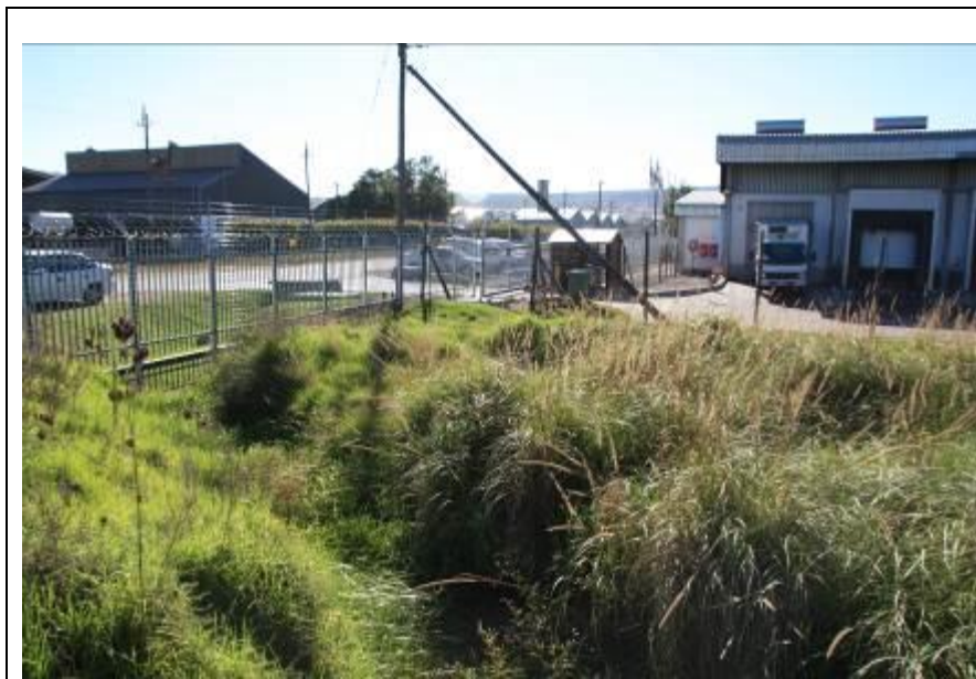
Figure 5a: Storm water drain 1 at southern fence
