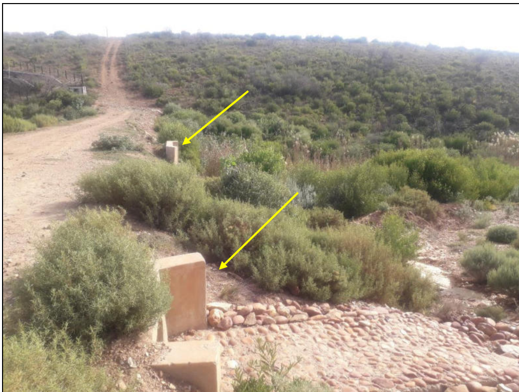
Photo 29: Larger dam – two culverts' outflows downstream
