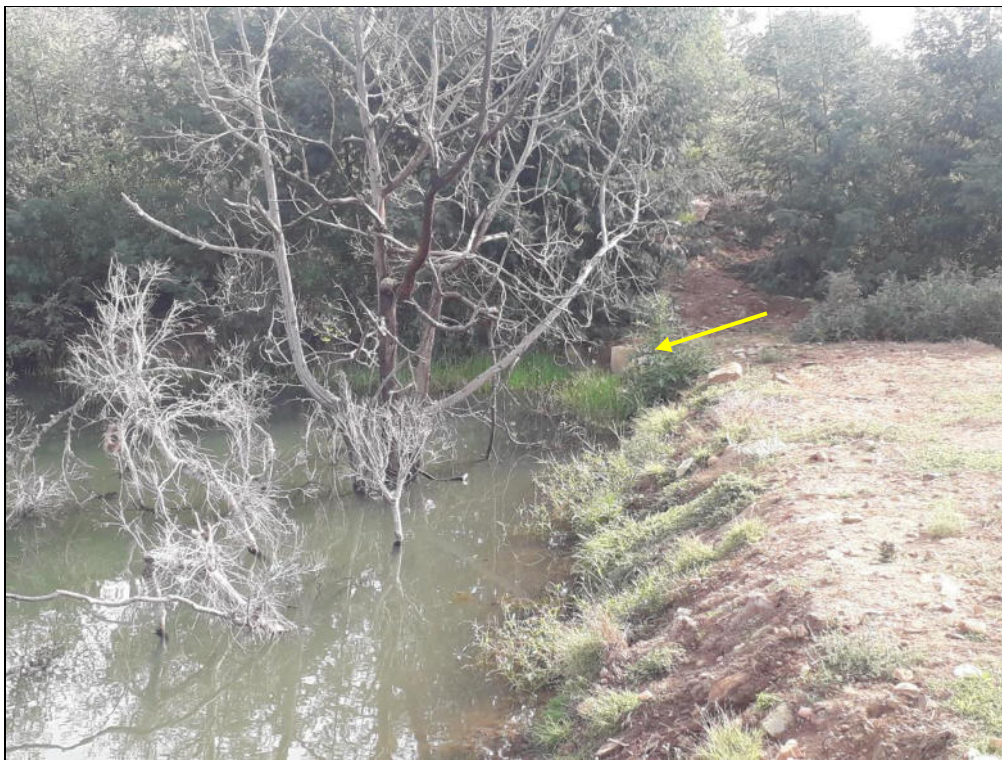
Photo 25: Small dam – note outflow culvert (indicated by yellow arrow)
