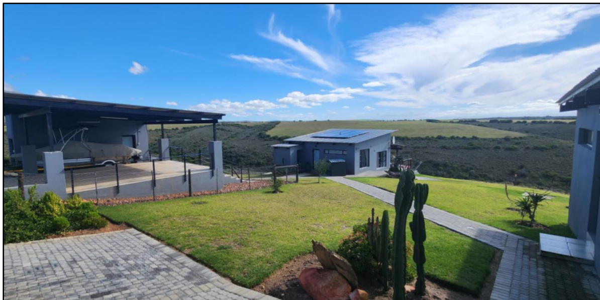
Photo 35: Two cottages and parking/utility building
