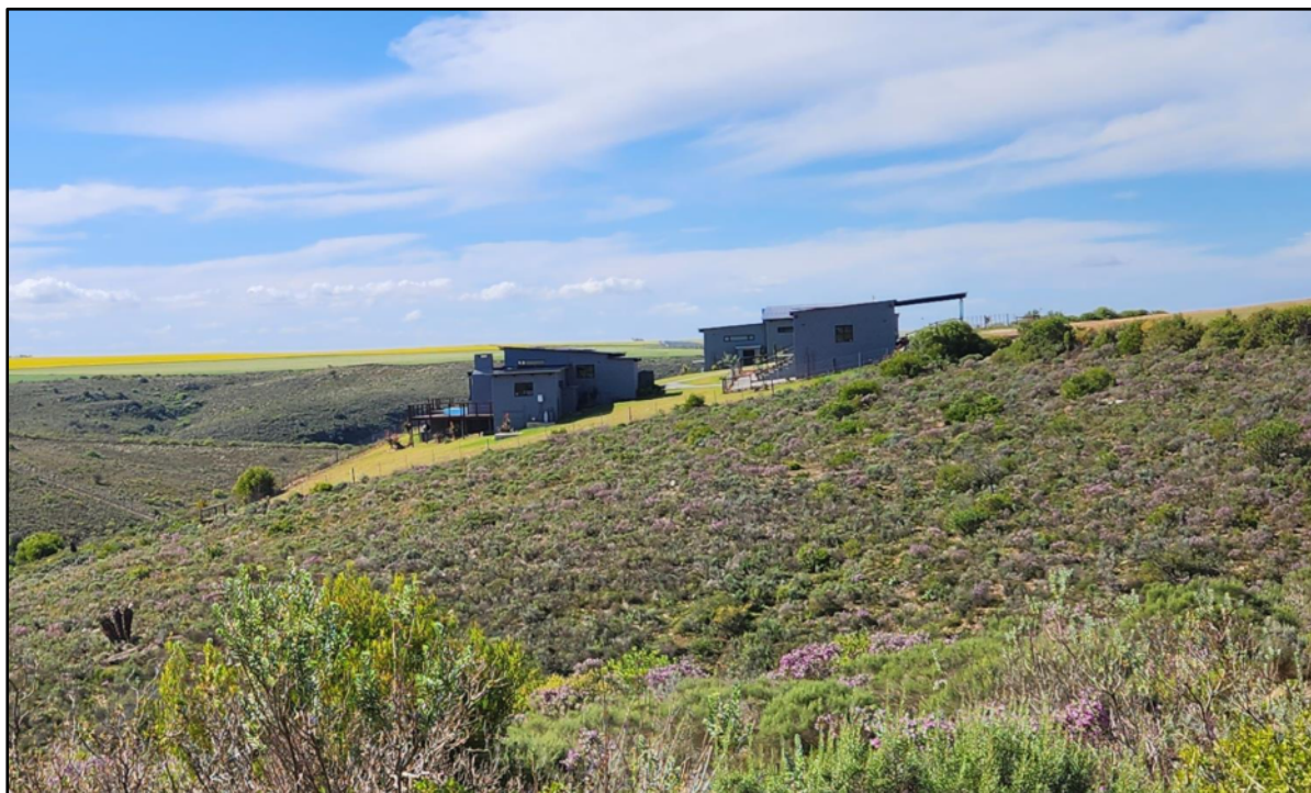
Photo 34: Two cottages and parking/utility building
