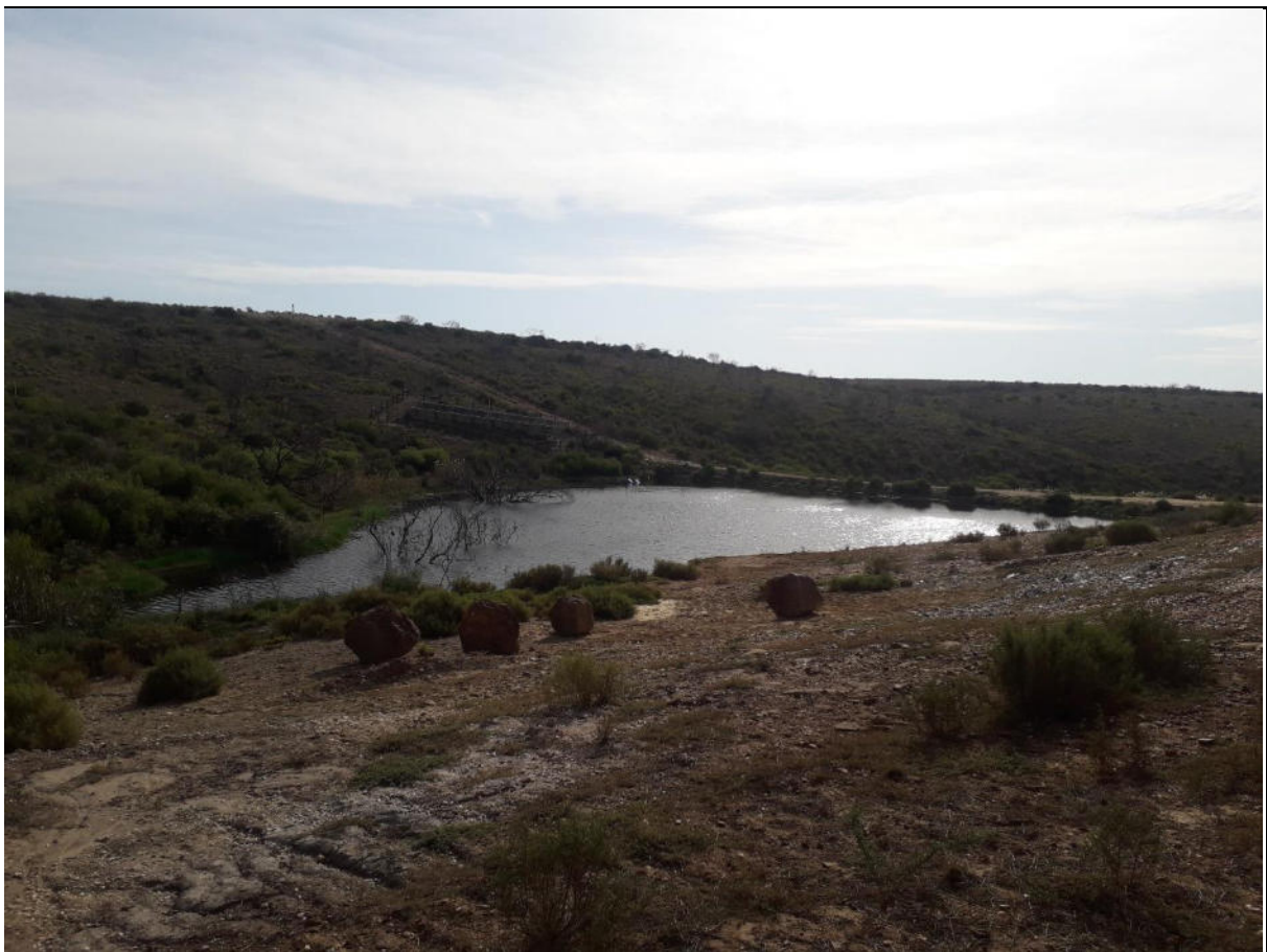
Photo 27: Larger downstream dam – looking North over dam
