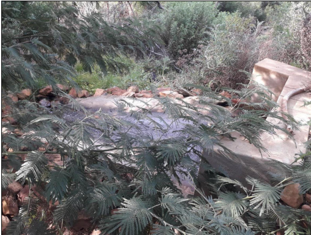
Photo 26: Small dam – outflow culvert downstream
