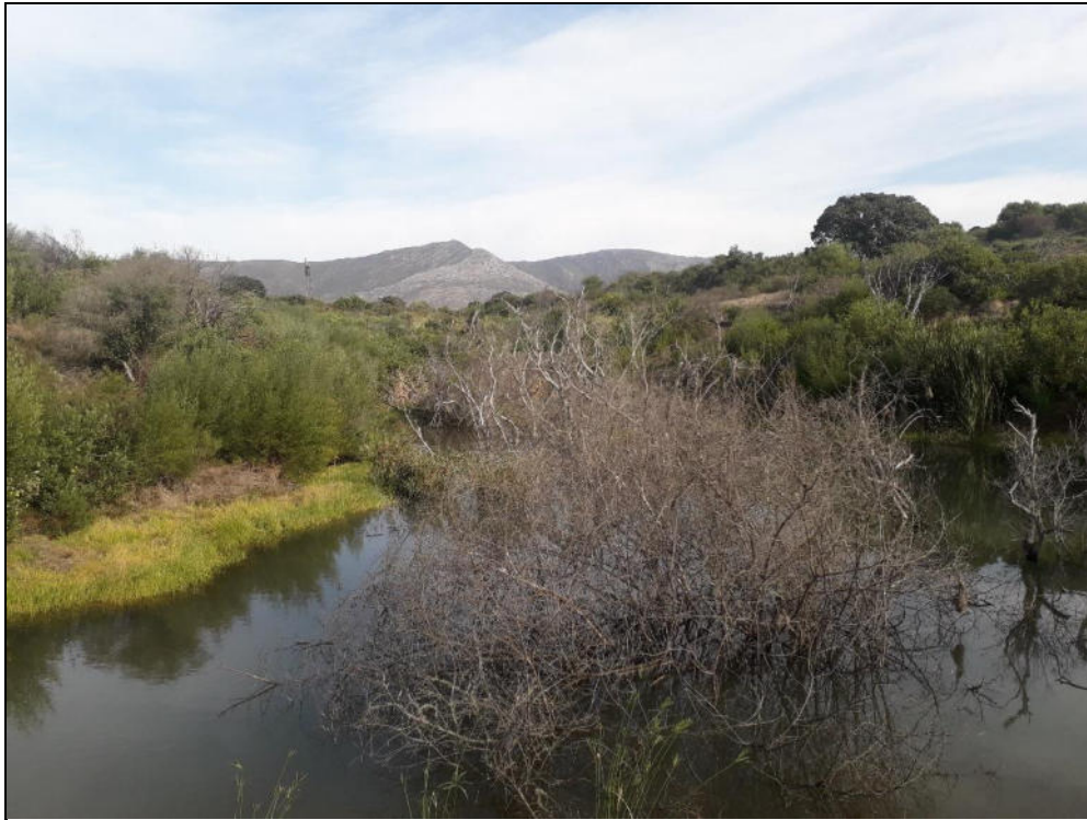
Photo 24: Small dam – looking South over dam
