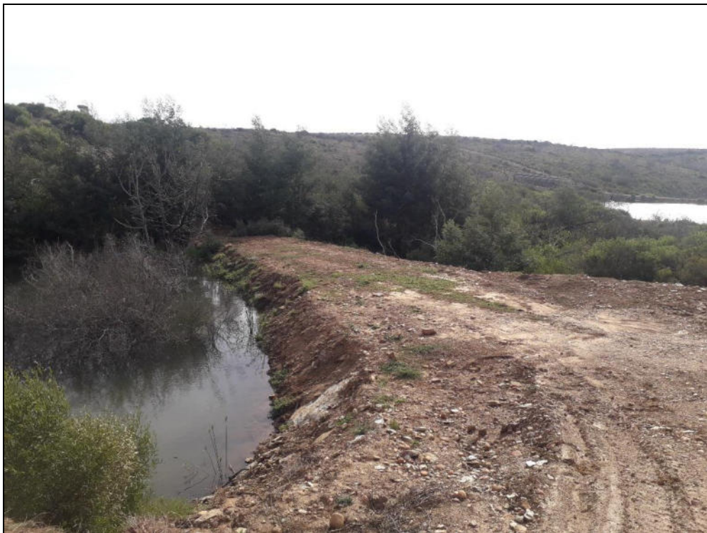
Photo 23: Small dam wall – looking West over damwall
