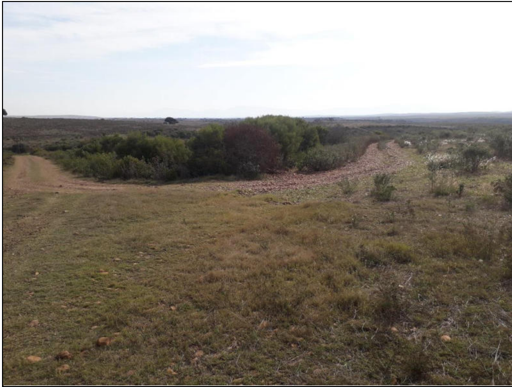
Photo 20: Road to Dams (looking northwest)
