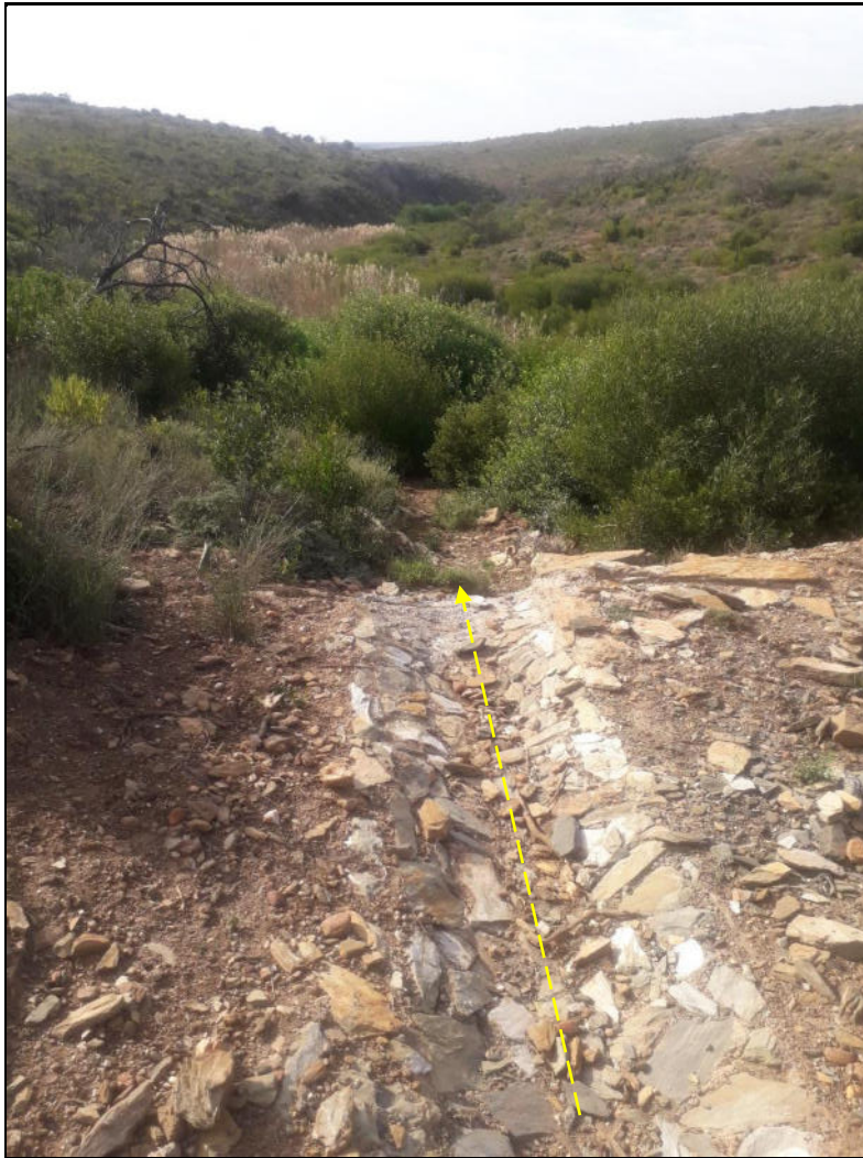
Photo 31: Larger dam – swale taking stormwater downstream from pumpstation area (yellow dashed arrow to indicate flow)
