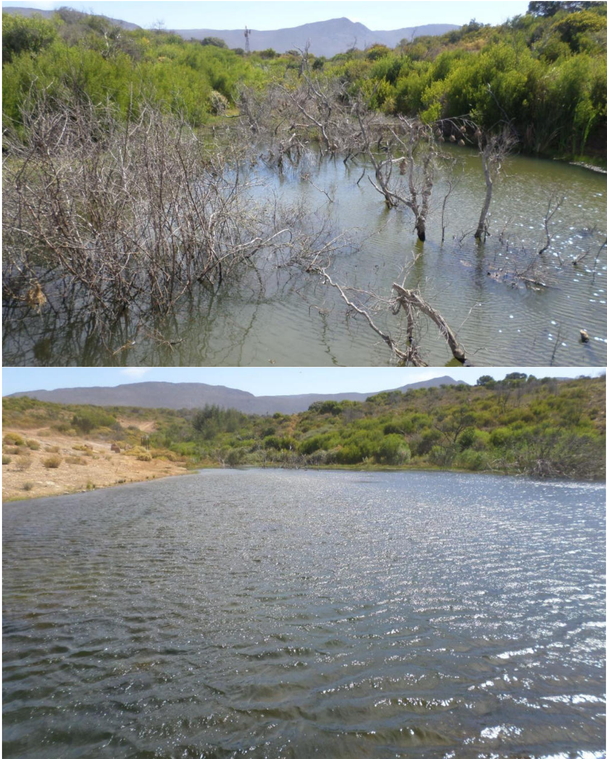
Figure 11. View of the upper (top) and lower (bottom) dams within the watercourse
