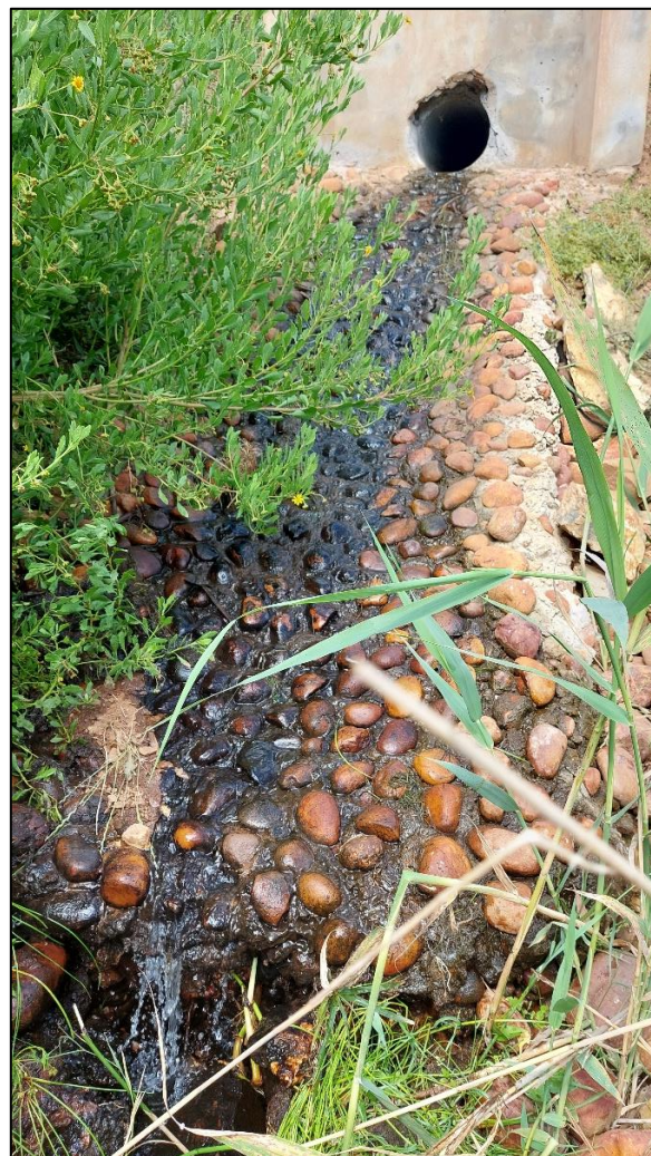
Figure 14: The outflow/overflow of the larger (lower dam). The flow measurements were taken at this location. Figure 13 indicate the location of this outflow/overflow (red dot no.2).
