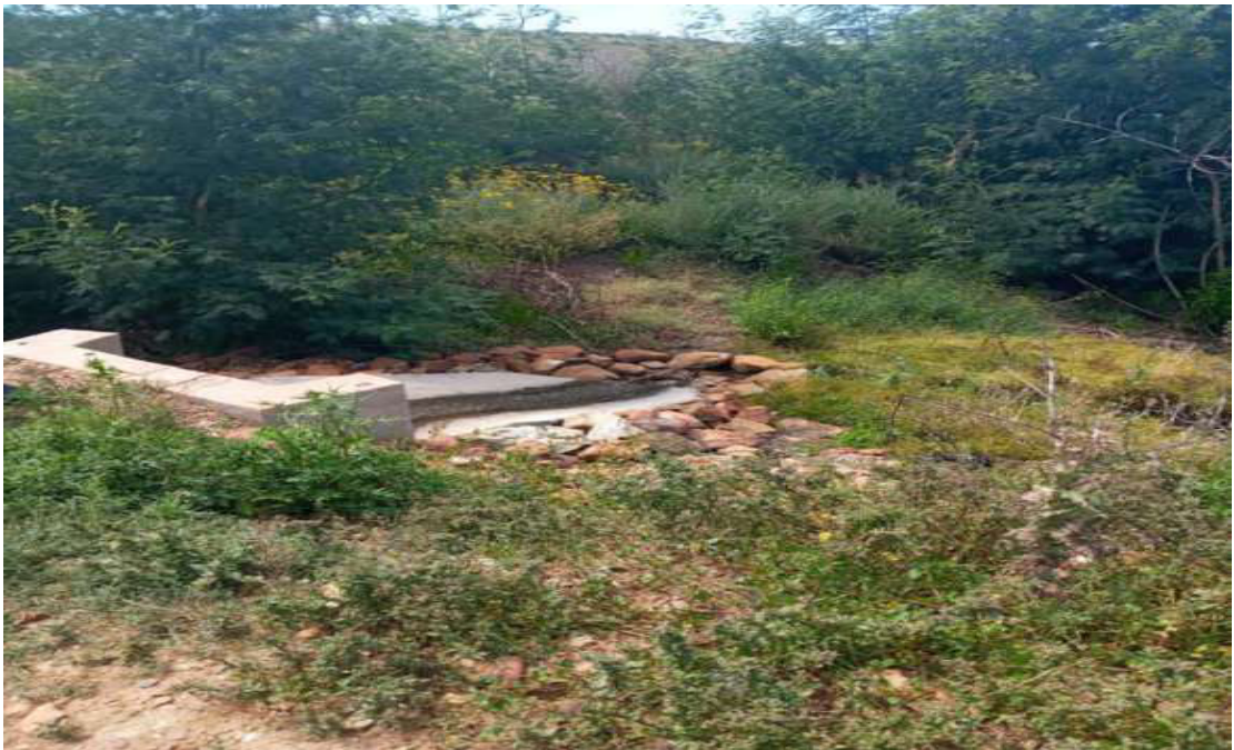
Photo 3: showing the culvert built through the dam wall to direct the flow in the water course
