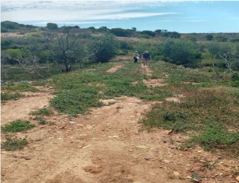
Photo 2: showing the Dam wall separating dam one and dam two.
