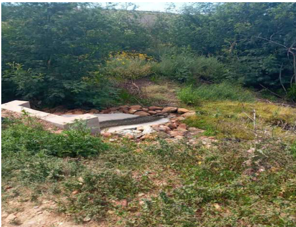
Photo 3: showing the culvert built through the dam wall to divert water.
