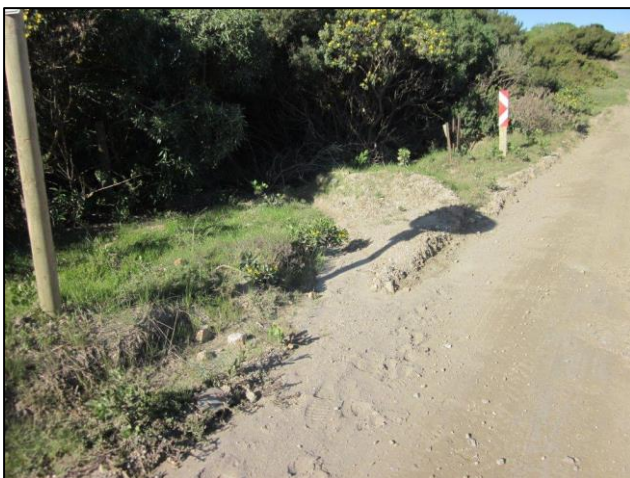
Photo 1 Dirt road to Cape Infanta, showing one of the stormwater “swales” carrying runoff from the road onto erf 134.
