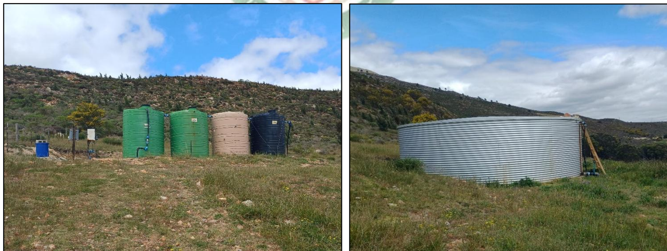
Figure 10: Images taken at BH03 of water treatment process. Left: Jojo tanks and dosing system. Right: Water Storage.
