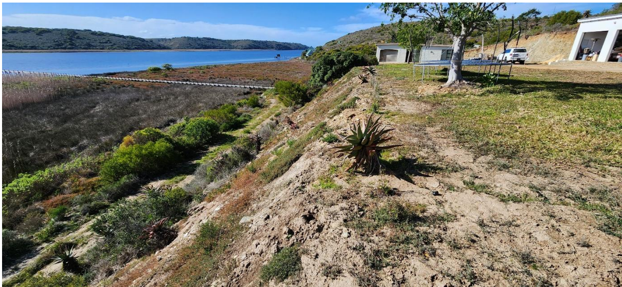
Photo 7: View of a portion of the cleared area around the main dwelling (facing southeast)
