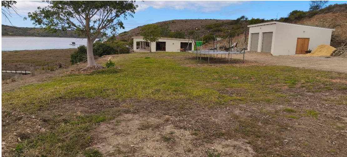
Plate 2: View (looking east) of cleared areas around original house (Footprint 1), with new garages in cutaway area on the right, and grass and planted, exotic Ficus trees on infilled area.
