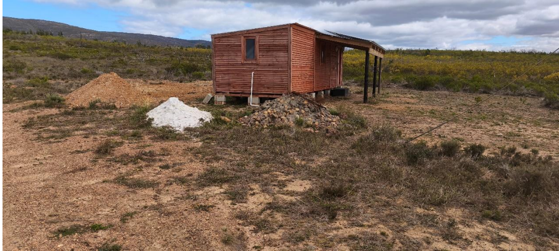
Plate 1: View of cleared areas around prefab house (Footprint 3), looking northwest.
