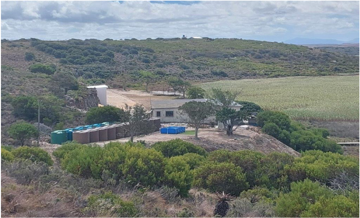
Photo 3: Visible clearing down the slopes of the site.
