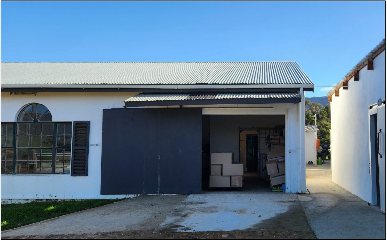
Photo 3: Loading are of the packing and store room. On is facing northwest.
