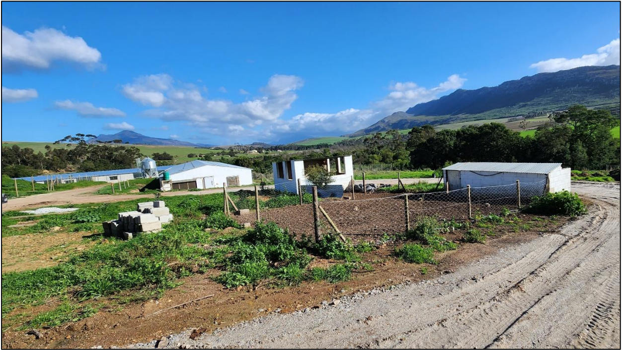
Photo 13: Facing northwest looking onto the pig pen area. In the background are houses 8 and 9.
