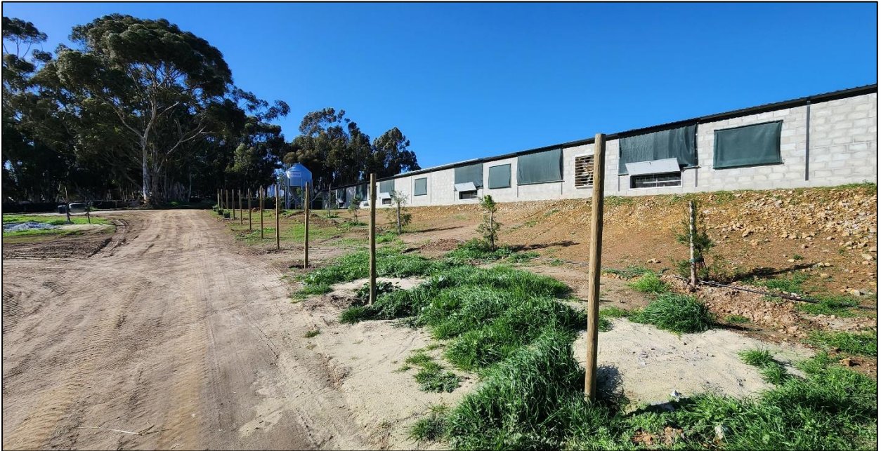
Photo 11: Chicken house 10, looking eastwards.
