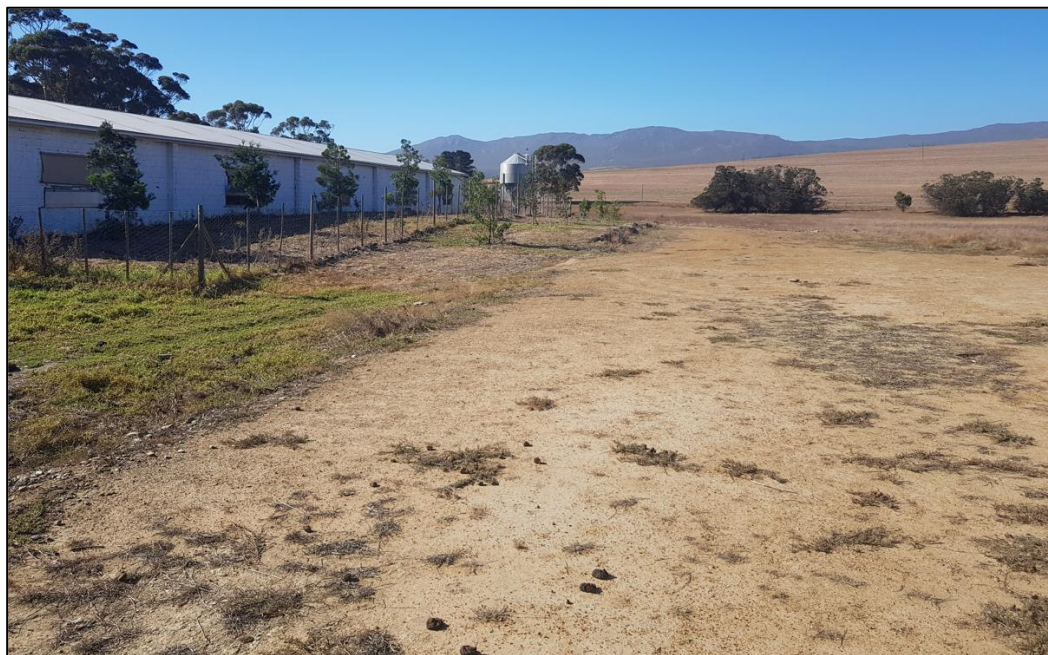
Figure 11: Disturbed land where houses were constructed. Image taken in 2019.
