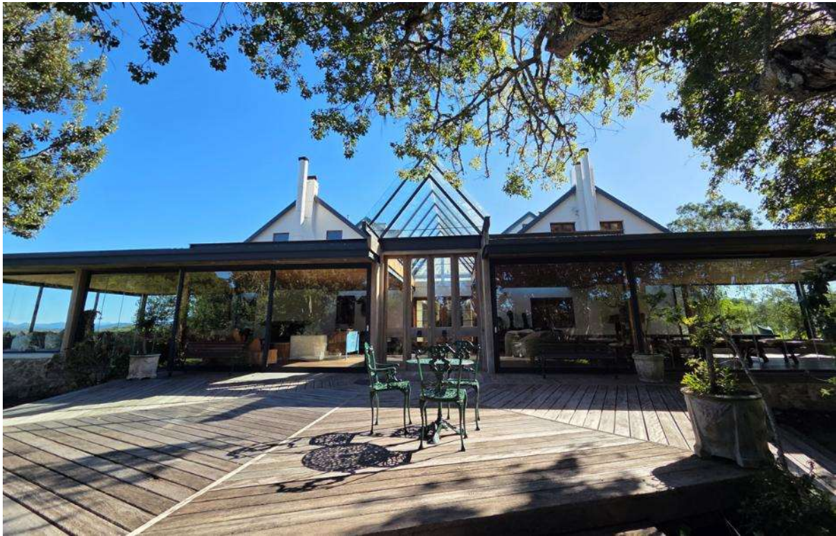
Photo 11: Southern façade: southern veranda floats with views of mountains and surrounding forest continuing. The original house and fabric clearly visible.
