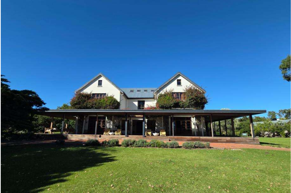
Photo 1: Northern facade showing the approved northern veranda wrapping around the dwelling.
