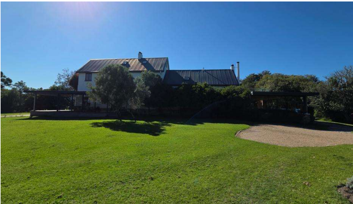
Photo 8: Western façade, on the left the northern veranda clip-on is light and hardly noticed. On the right is the approved enclosed southern veranda clip on.
