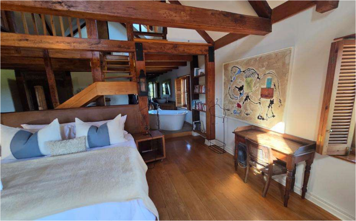
Photo 28: 1 st Floor, west wing existing master bedroom's bathroom, to be converted.
