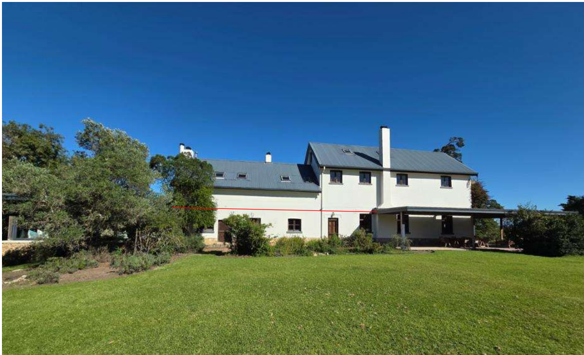
Photo 14: Southern veranda to wrap around onto the eastern façade in similar fashion than the precedent set with the northern wrapping veranda and to join the northern veranda. Red outline depicts the approx. line of a new open veranda, to clip onto the original building, allowing separation with lightweight floating wood structure (refer to architectural drawings).
