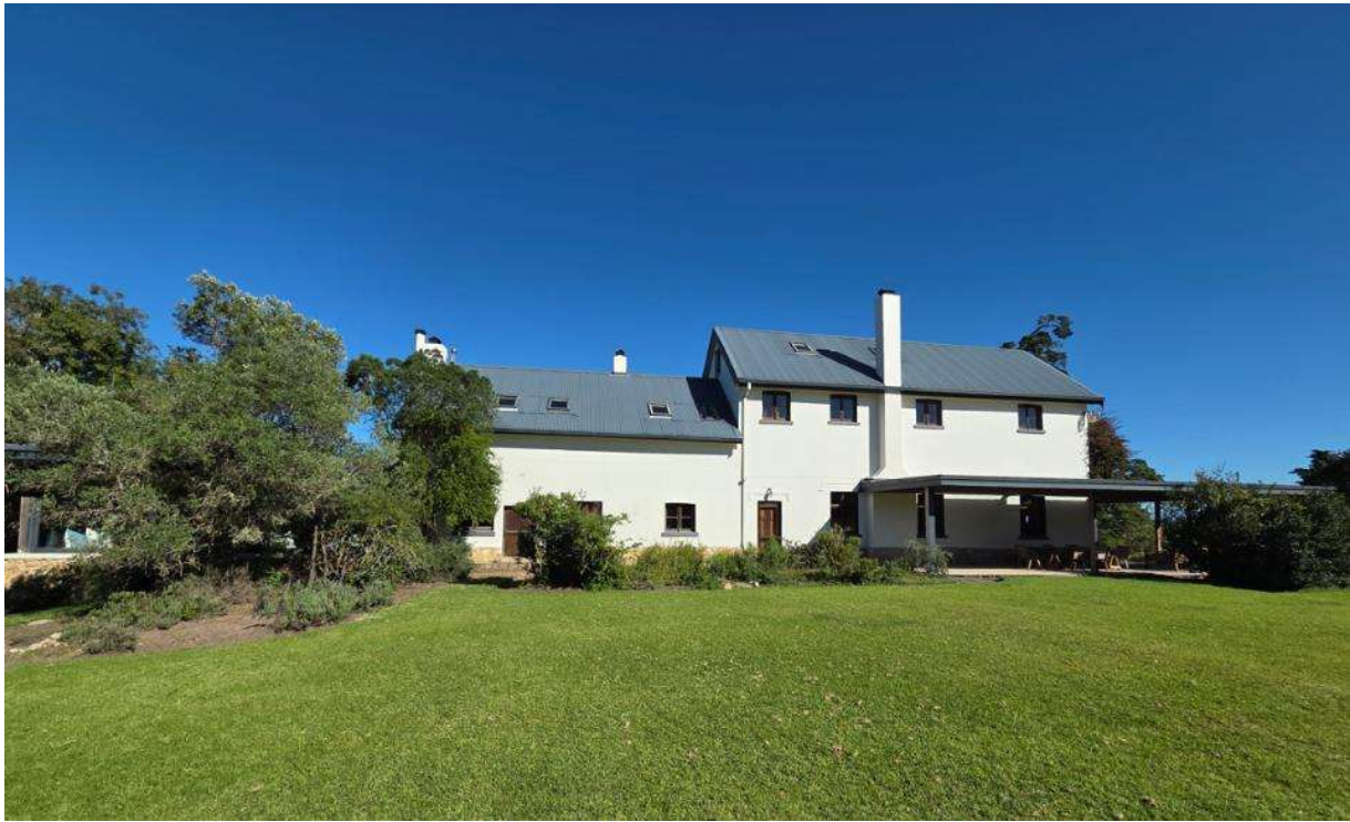
Photo 13: Eastern façade, on left southern enclosed veranda slightly visible amongst the trees, northern wrapping veranda visible on the right.
