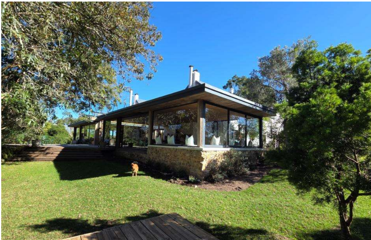
Photo 12: View from the southeastern side of the southern enclosed veranda.
