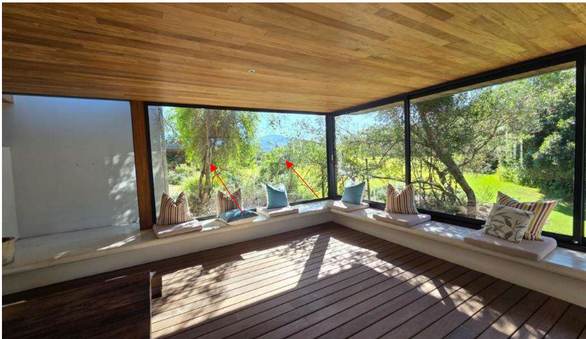
Photo 25: Extension of the southern veranda (east wing) by adding a wrapping component onto the eastern façade, separated by a sliding glass door. The component will lead onto an open veranda similar to the northern veranda precedent with a skylight separating the old and the new.
