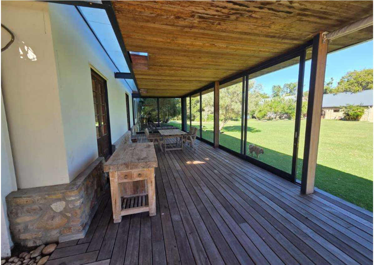
Photo 7: Northern veranda wrapping on the western façade, note the separation skylight from the original building and large framed glass sliding doors to cut off coastal winds to allow outdoor living.
