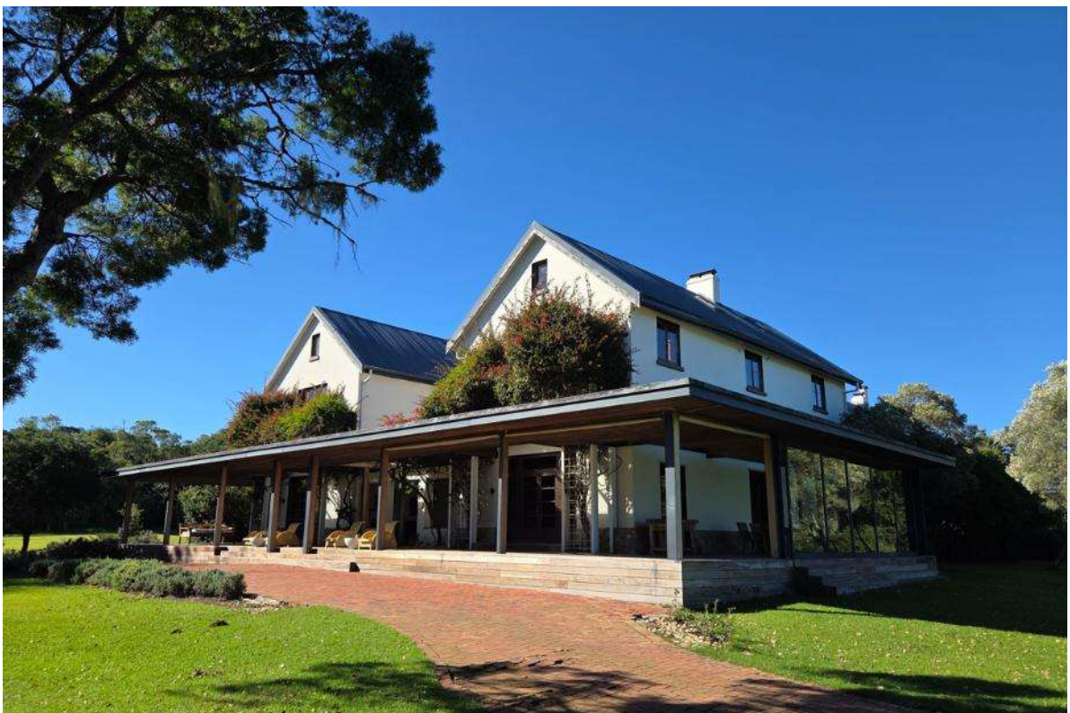
Photo 2: View from the northwest showing the approved northern veranda wrapping partly onto the western elevation.
