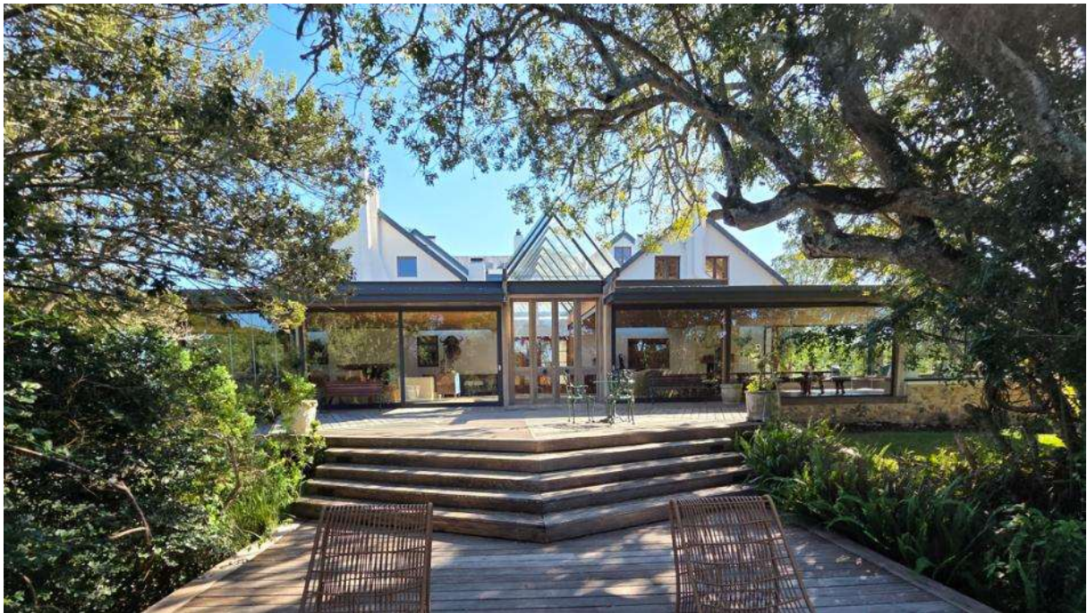
Photo 10: Southern façade, original main house visible through the glass clip on, light filters between closed veranda roof and original house walls due to separation.
