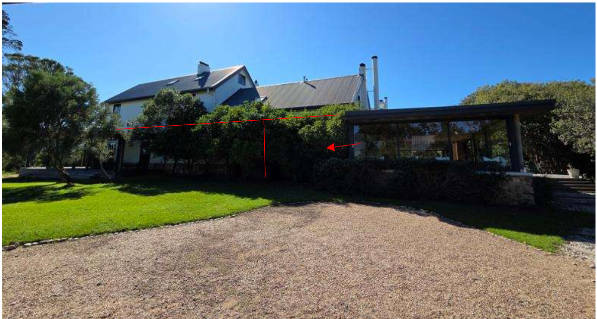
Photo 16: Southern veranda to wrap around onto the western façade and connect with the northern veranda. Red outline depicts the approx. extent of the new veranda which will largely be open except for the kitchen extension which will be glassed as per the existing precedent set. The veranda will clip onto the original building, allowing separation with a lightweight floating wood structure (refer to architectural drawings).
