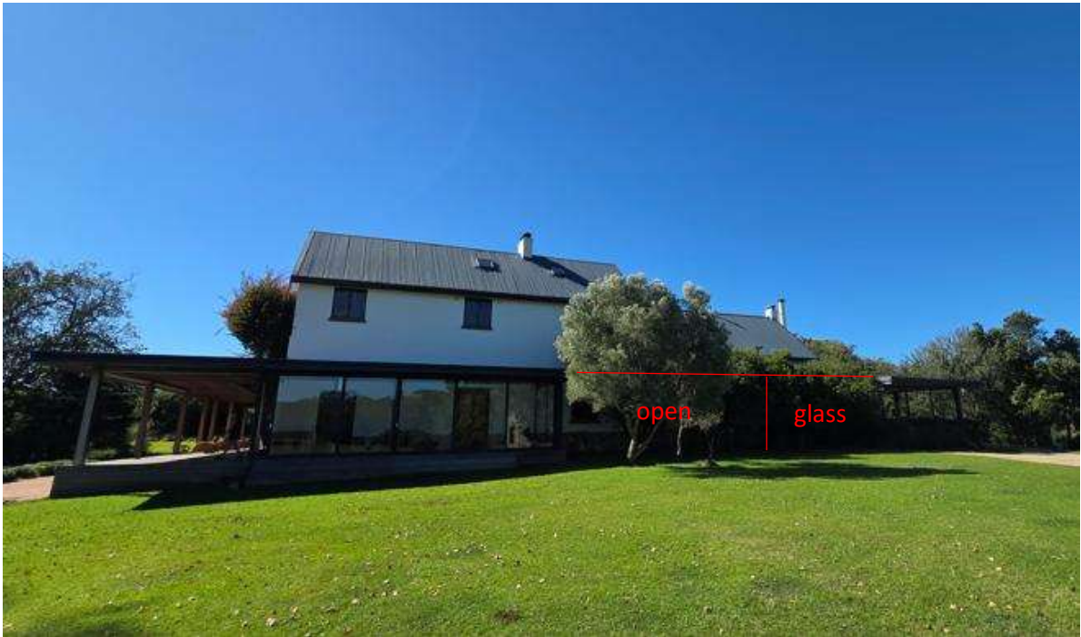
Photo 17: Southern veranda to wrap around onto the western façade and connect with the northern veranda. Red outline depicts the approx. extent of a veranda (largely open besides the kitchen section which will be glassed), to clip onto the original building, allowing separation with lightweight floating wood structure (refer to architectural drawings).
