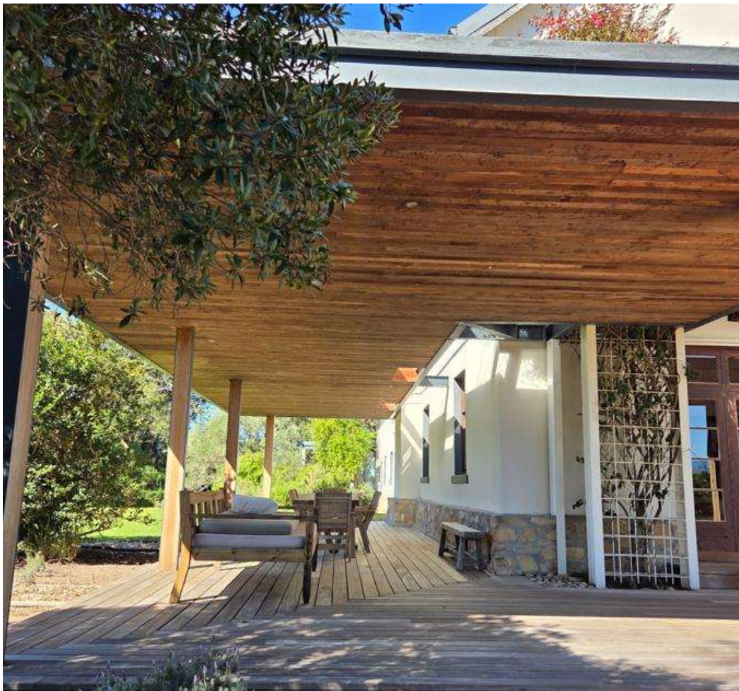
Photo 4: View from the northern façade showing the wrapping veranda on the east, note the separation skylight from the historic building by allowing the new structure to clip onto the old and to separate it from the historic dwelling by allowing light to come through.
