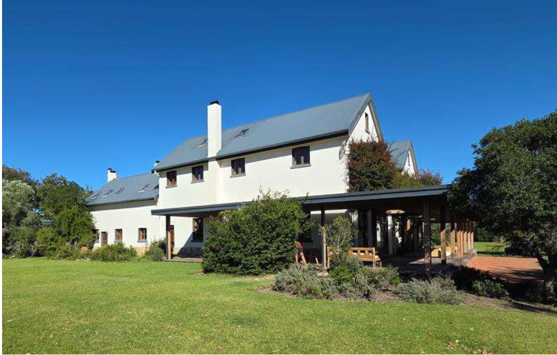
Photo 3: View from the eastern façade, showing the approved northern veranda wrapping around the dwelling.
