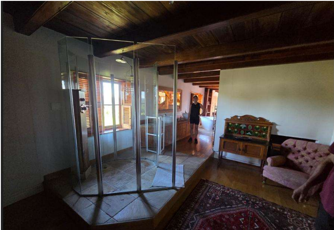
Photo 30: Current bathroom of the master bedroom to be reconfigured.
