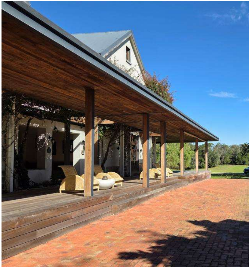
Photo 5: The same effect as shown in Photo 4, the northern veranda clipped onto the building, creating a free-standing impression by allowing light to come through separating the new and the old structure accentuating the old building features.
