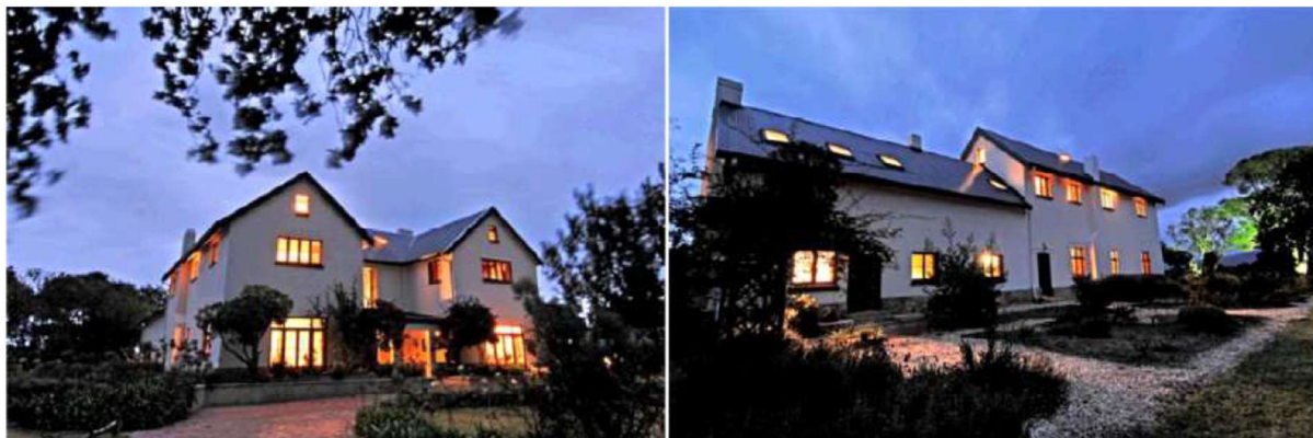
FIGURES 12a & 12b: Forest Hall after the second round of repairs, structural stabilization measures and addition of the new loft accommodation by former owner Michael Johnson (note the skylights along the roof faces). The house's characteristic stucco and wall creepers had to be removed in order to carry out the work. The external walls are currently plastered and painted. (Photo: Jacobs, 2010)
