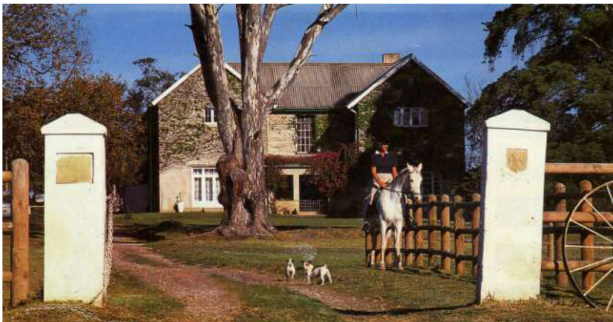
Figure 10: Forest Hall in 1990 after restoration by Hilary Newdigate Peter (mounted on the horse in the foreground). The hall window above the central entrance porch has been enlarged (though this was probably done before her time) and wall creepers re-grown. The casement windows are by now likely to be substantial, if not complete replacements given the condition of the house prior to 1971 (refer Figure 8). (Photo: Jacobs, 2010)
