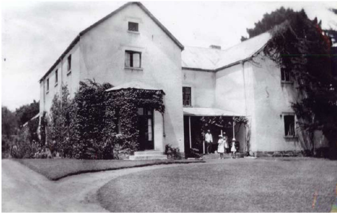
Figure 6: Early photograph of the exterior of Forest Hall. This photo appears to have been taken during the mid-1920's judging by the style of clothing worn by the figures in the foreground (presumably members of the Newdigate family). Note the small relative sizes of the windows, which are inward opening casements with shallow arched upper panes typical of a fashionable rural English country gentleman's residence of the period. The stepped Gothic Revival drip mouldings are the only decoration in an otherwise austere façade. The central porch is supported on four (what appear to be) cast iron columns. The corrugated iron roof may already be a replacement (compare with Figure 5 ). The only element still surviving on the current façade today, is the front door. All other elements including the bay window, casements windows, roof sheets and veranda colonnade have either been removed or replaced. Note the 's'-shaped wrought iron wall anchor bracket on the right-hand wing, suggesting that even at that stage, there were structural problems with at least this external wall. (Photo: Jacobs, 2010)
