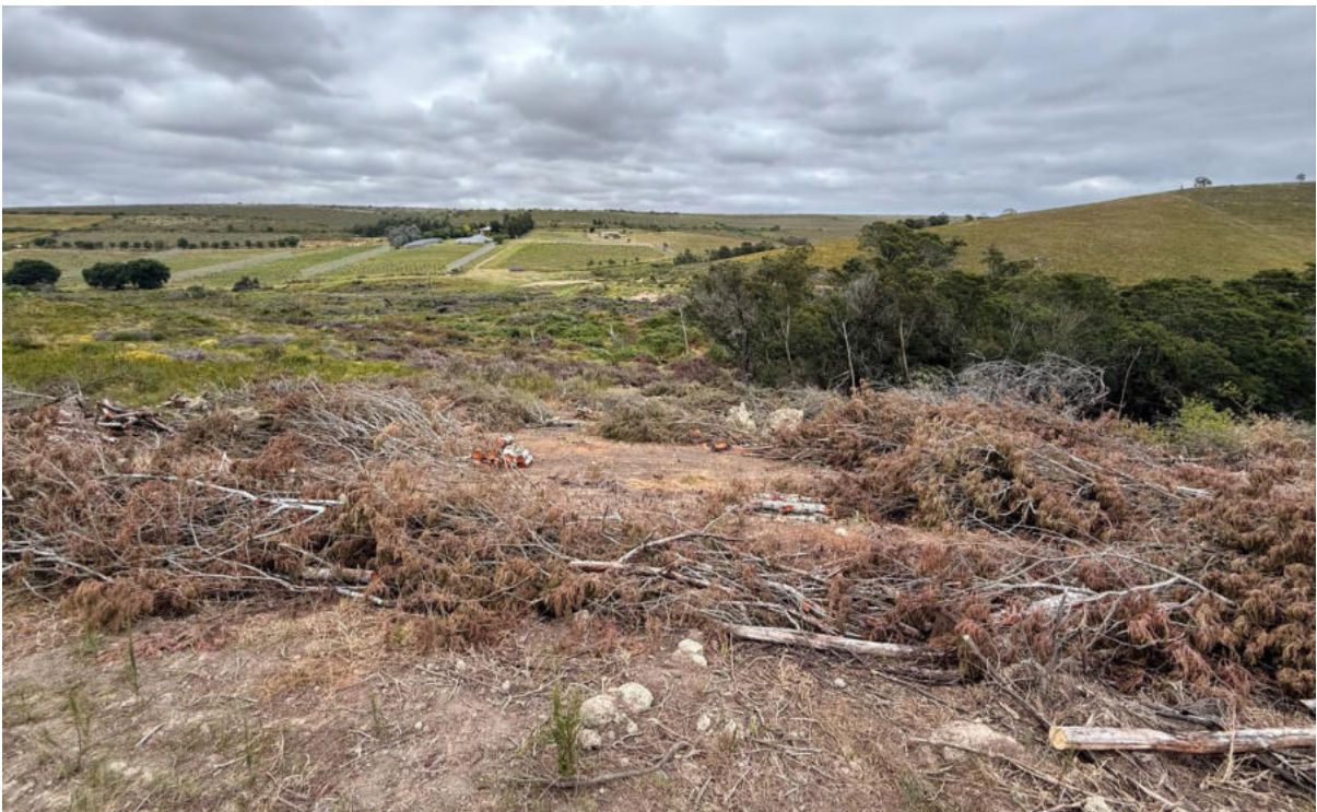
Figure 44: Clearing activities of Black Wattle trees is on-going at the project site. The dense stands of these invasive trees are a major disturbance at the project site (Photo: Colville & Cohen, 2025).
