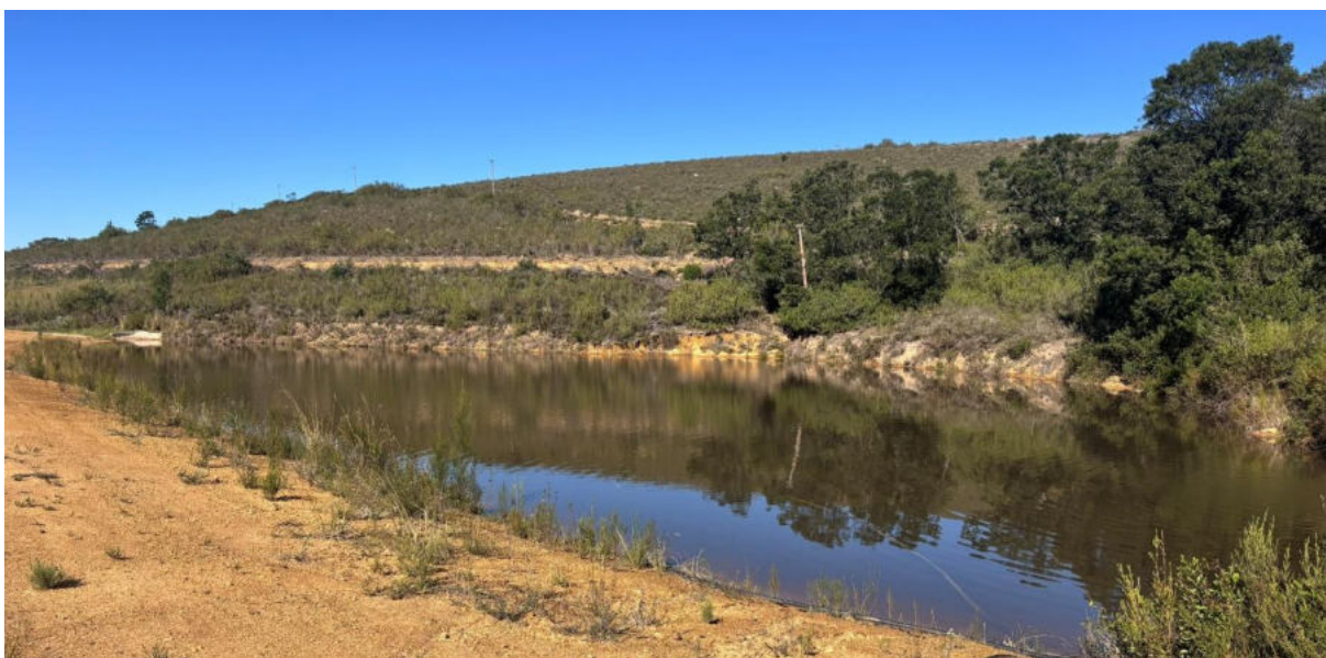
Earth dam on eastern boundary of Ptn 3/186
