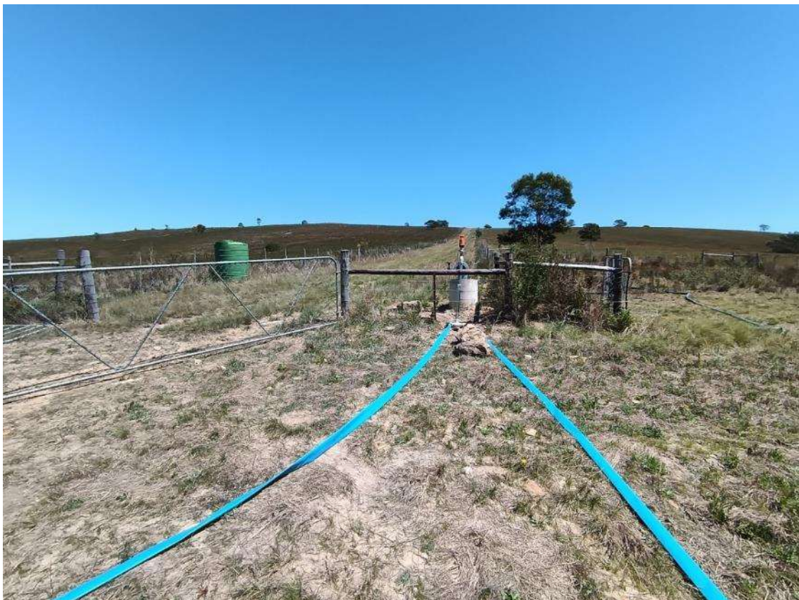
Figure 16: Looking north-west from the road in the middle of Pocket 4 where water is pumped to the top of the hill.
