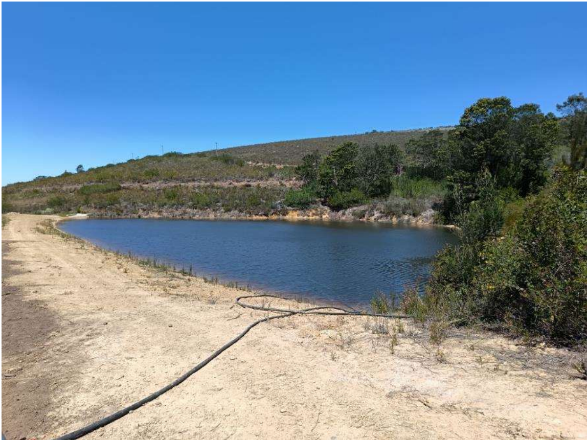
Figure 3: Showing a small existing Dam at the entrance to the property on the southern boundary.
