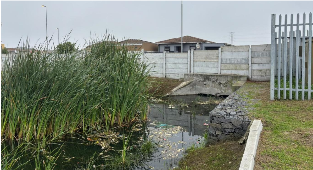
Photo 12: Stormwater pond that serves as the designated wetland offset area to compensate for impacts on Wetland 7. The inlet from the underground piped section of Wetland 7 is visible on the left-hand side of the pond.
