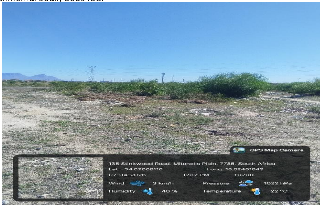
Photo 2: Wetland 7 with extensive invasion by alien vegetation. While partial piping was approved, an independent environmental audit confirmed that the wetland was piped beyond the approved scope.
