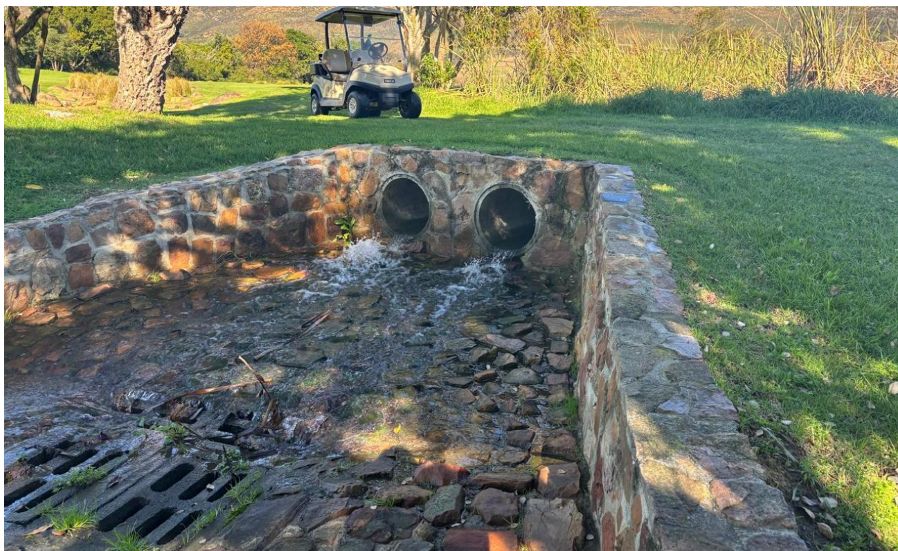
Figure 19: Infrastructure where a portion of the artificial channel enters an underground pipe (downstream of Dam 2).
